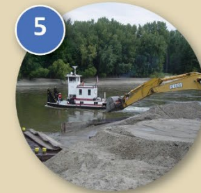
5 Vernon Avenue Dredge Material Management Site
