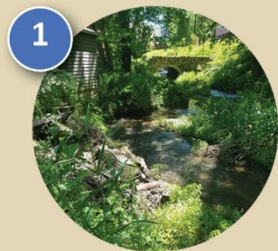
1 Spring Creek Site Stabilization
