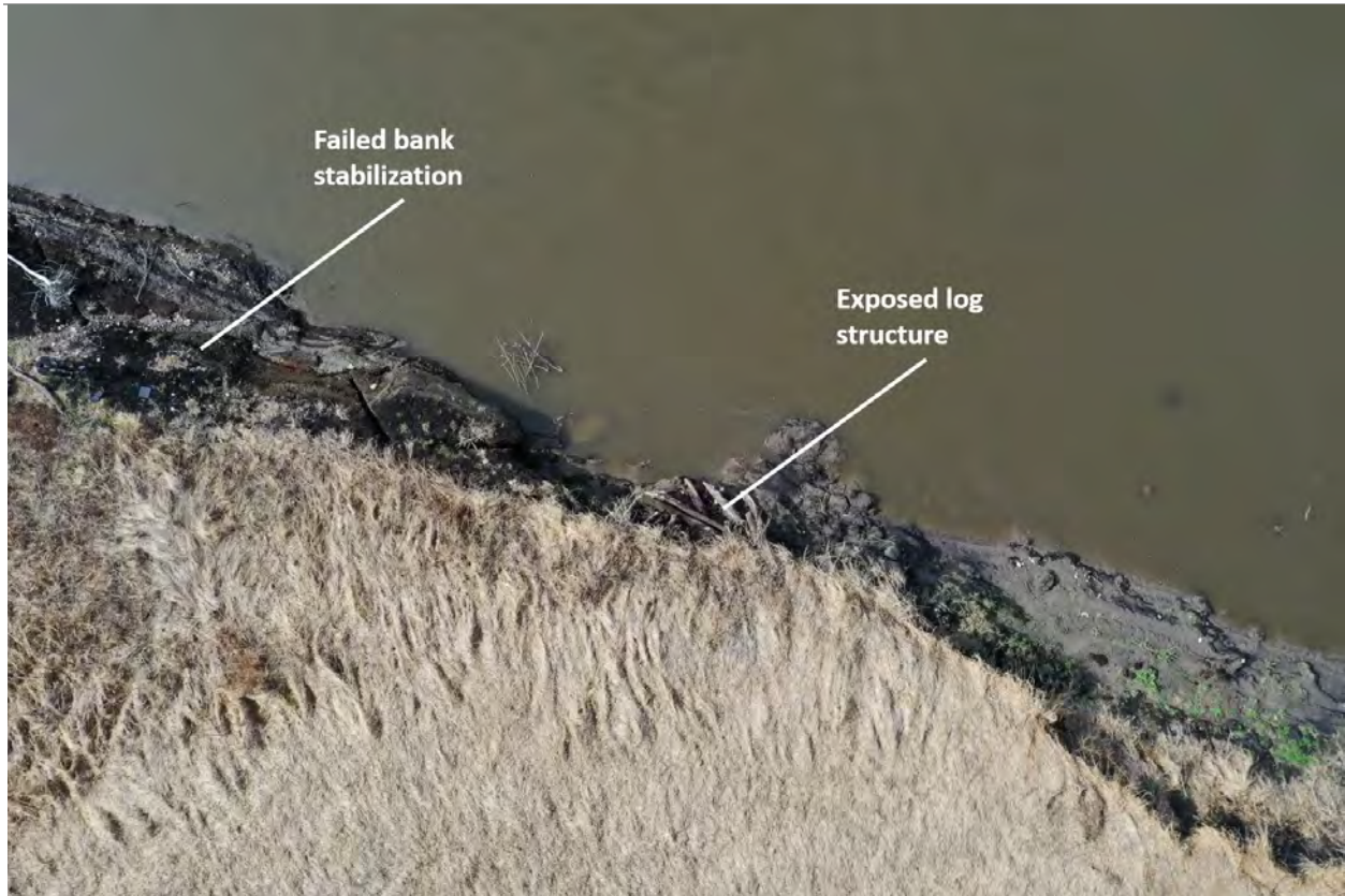
Figure 4: Drone image showing exposed log crib structure and failed bank stabilization.
