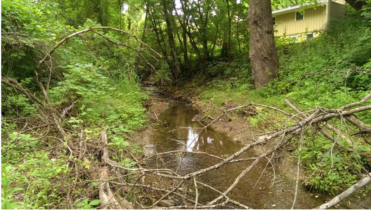
Photo 1: Upstream section unaffected by significant stream bank instability. Structure is approximately 50-feet from the channel.
