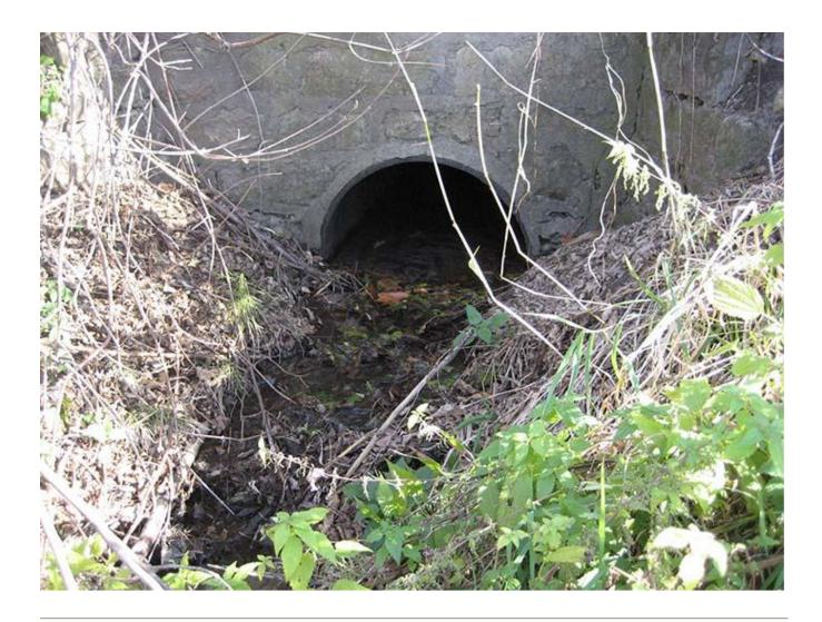
Moderate erosion on sides of culvert.
