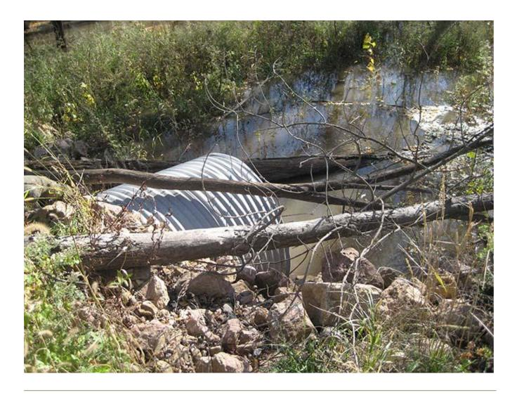
Small amount of erosion on riverside of trail at metal culvert.
