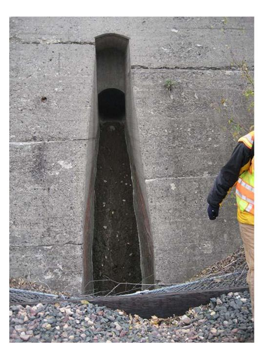
Lower side of culvert; minimal erosion; lots of rock surrounding the culvert.
