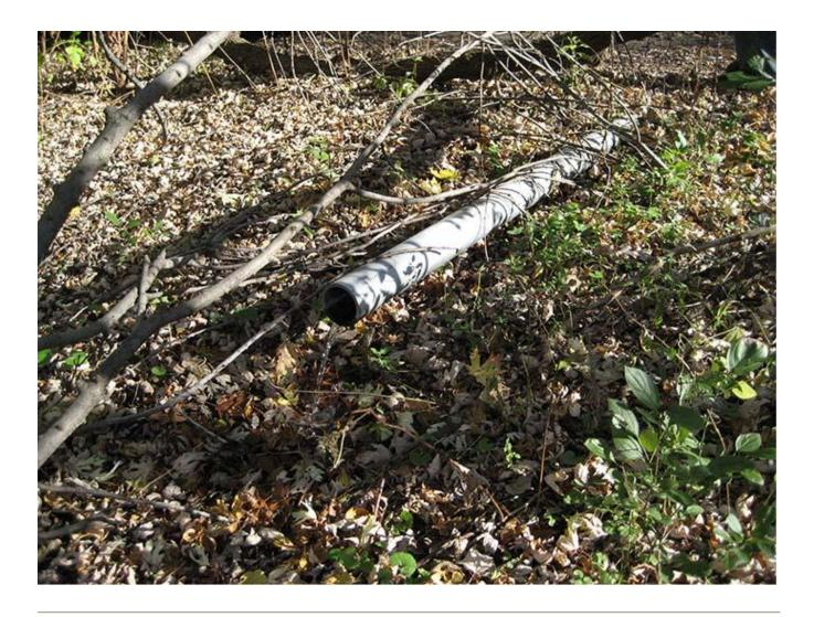
Major erosion due to outlet of PVC pipe.
