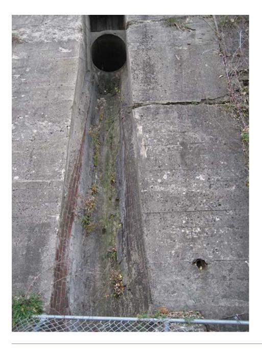
Culvert on lower side of railroad tracks; sides of culvert starting to erode; minimal erosion.
