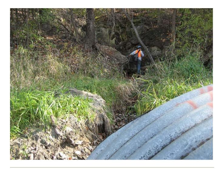
Down slope side of culvert in picture #1; starting to erode.
