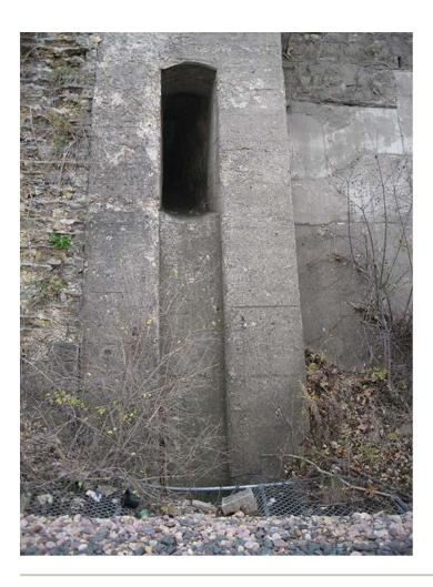
Lower side of railroad tracks; culvert had lots of rip-rap; sides starting to erode; moderate erosion.
