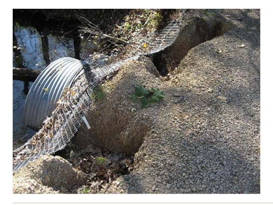
Newly installed metal culvert, matting and fencing laid over slope to control erosion; some major erosion on trail.
