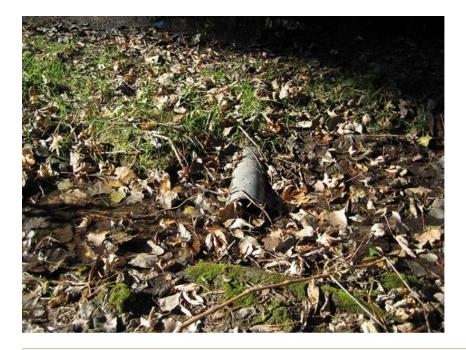
PVC pipe going under trail; pooling water at top part of pipe; possibly clogged; minor erosion; approx. 20-feet between pipe shown in pictu
