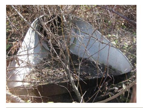
Culvert on river side of trail; cement slab under lip of culvert then approx. 6" drop-off to ground; lots of logs and debris at bottom.
