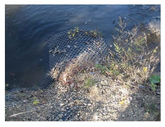
Newly installed metal culvert, matting and fencing laid over slope to control erosion; some major erosion on trail.
