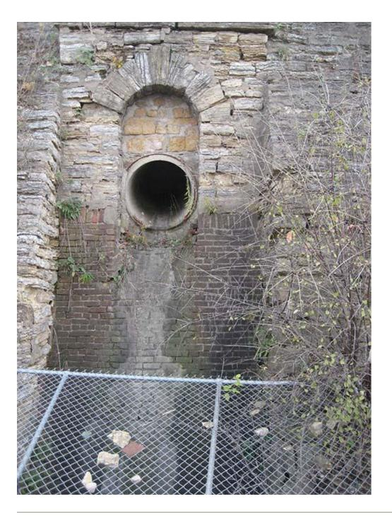
Lower side of culvert; full of rock and sand; water pooling at outlet; minimal erosion.
