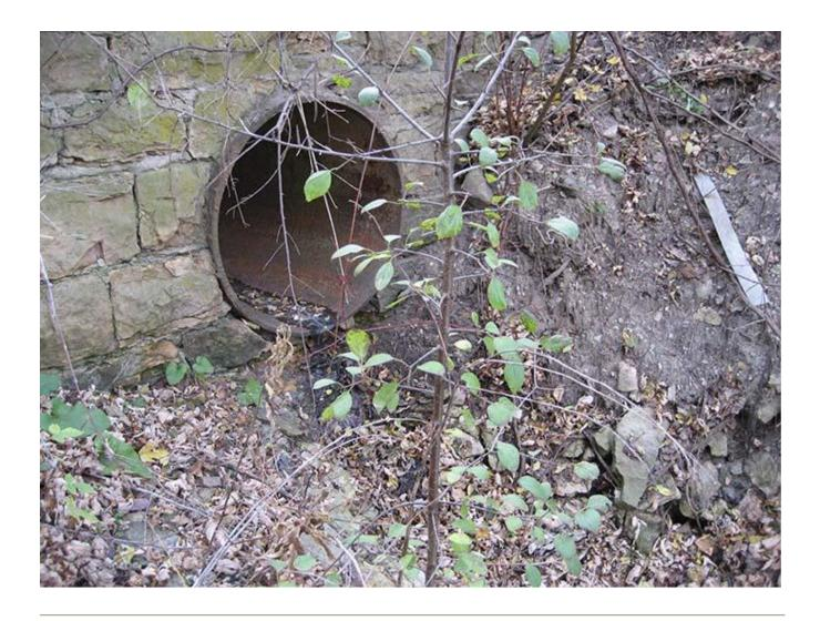
Major erosion; sides cut out all the way to the river; loose rock and exposed soil.
