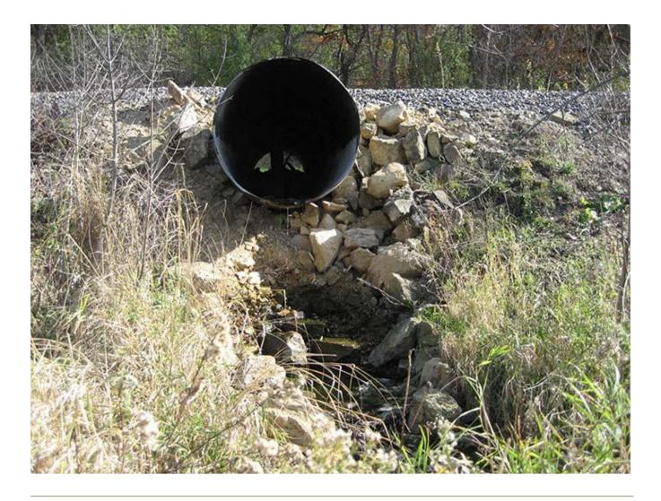
Down slope side of culvert in picture #1; starting to erode.
