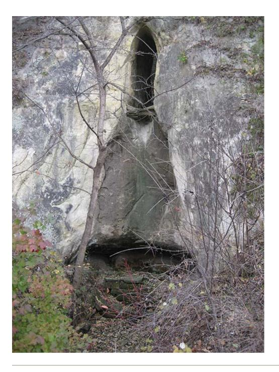
Major erosion on lower side of railroad tracks; undercutting bank.
