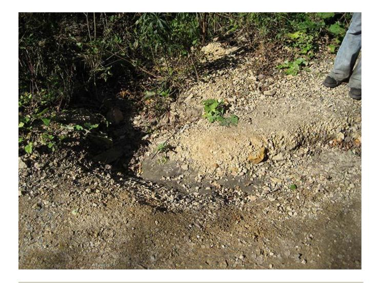
Erosion of trail due to no culvert going under trail; major erosion.
