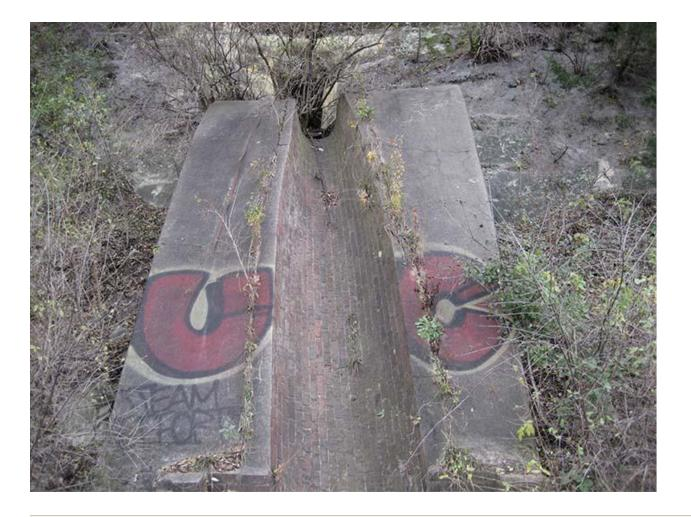
Lower side of culvert; lots of large rock and rip-rap protecting river bank; minimal erosion.
