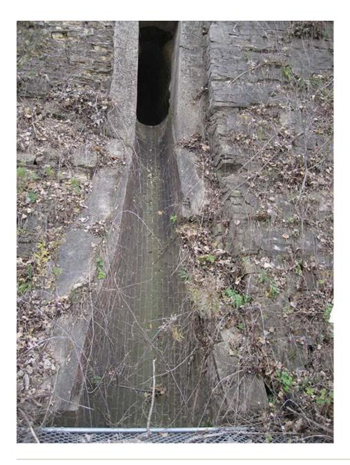
Lower side of railroad tracks; sides of culvert starting to erode; minimal to moderate erosion.
