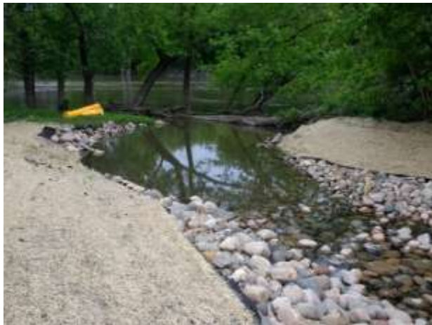
Looking North toward MN River
