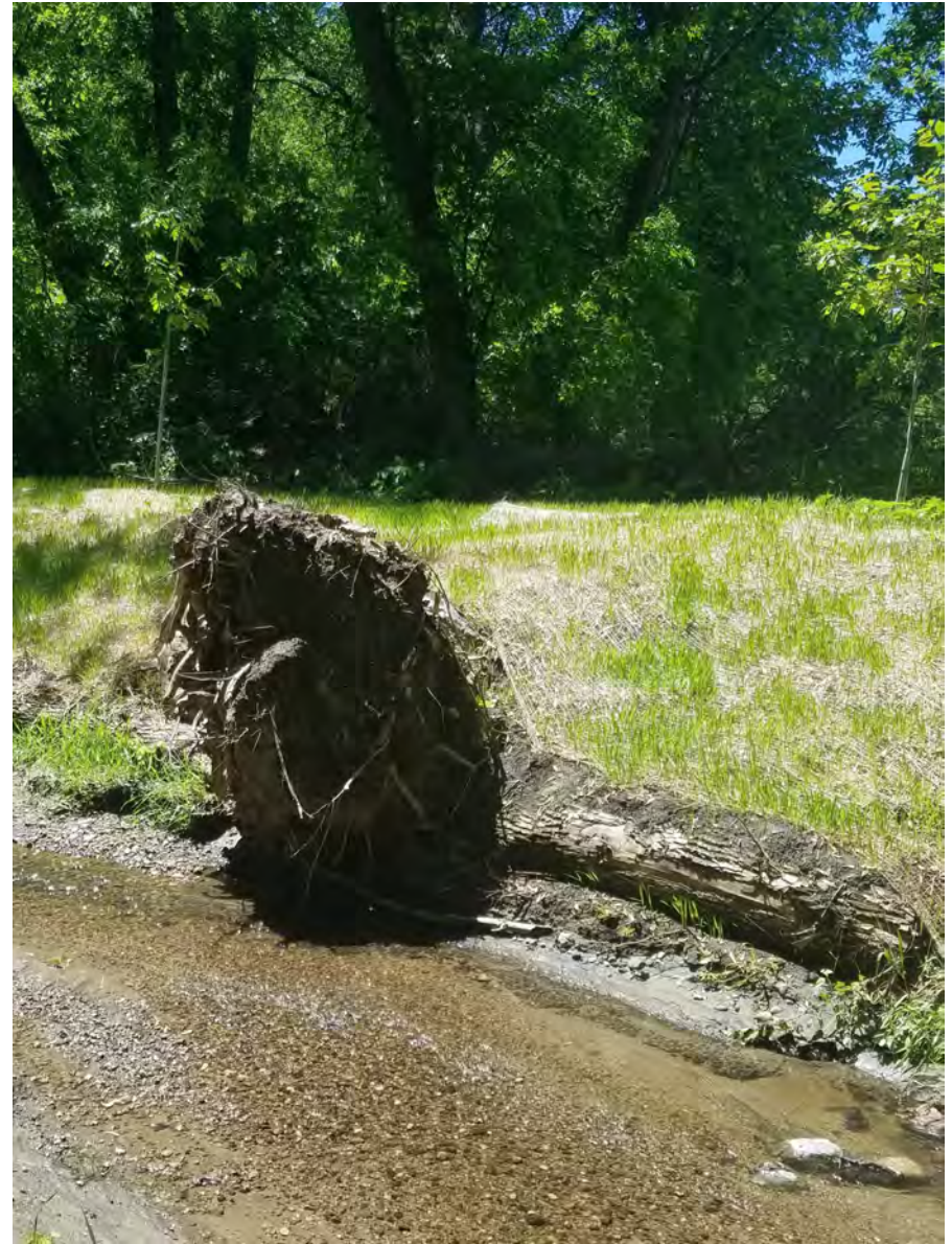
May 28, 2021—Right bank re-graded and additional stabilization/erosion control measures installed. Trees planted on upper right bank.
