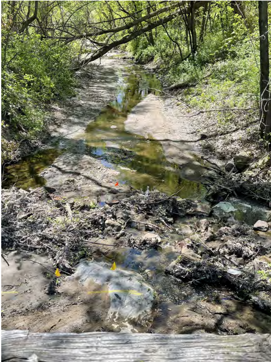
May 7, 2021—View downstream from Crosstown Boulevard bridge with utility locations (yellow = gas, orange = fiber optic), prior to construction.
