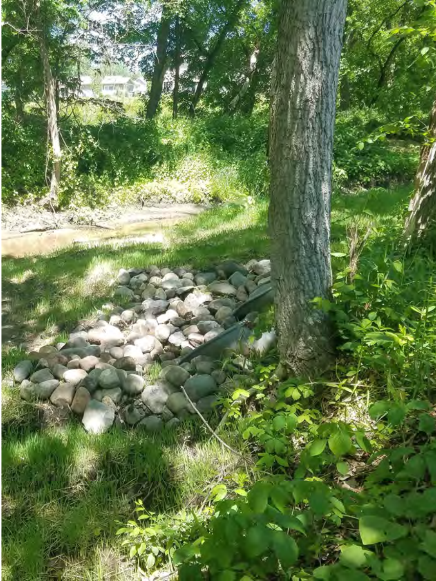
May 28, 2021—Additional riprap placed.
