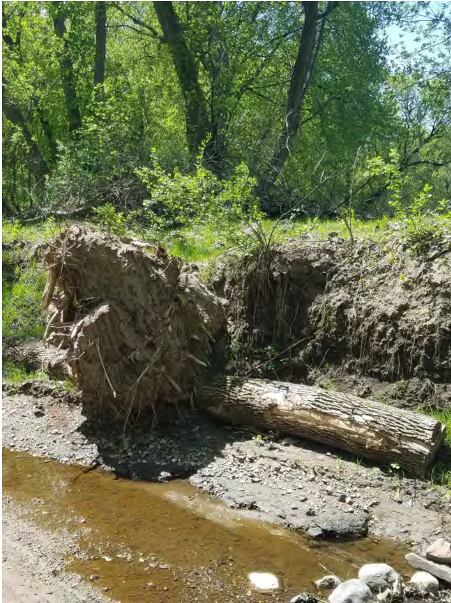
May 6, 2021—Right bank rootwad and vertical bank.
