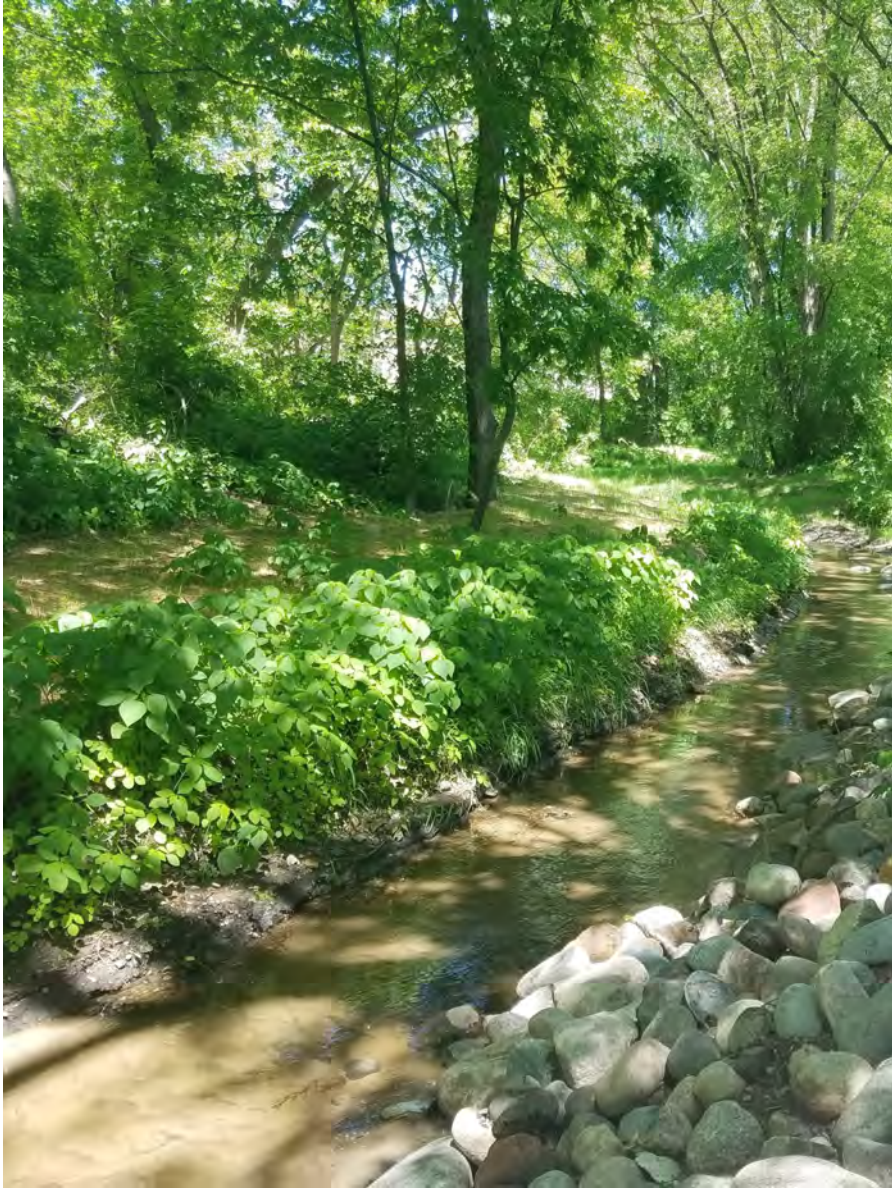
May 28, 2021—Looking upstream at additional grading and erosion control measures placed on right bank.
