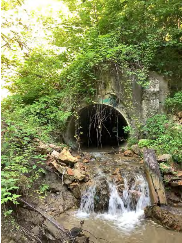
Frontal view of outlet pipe
