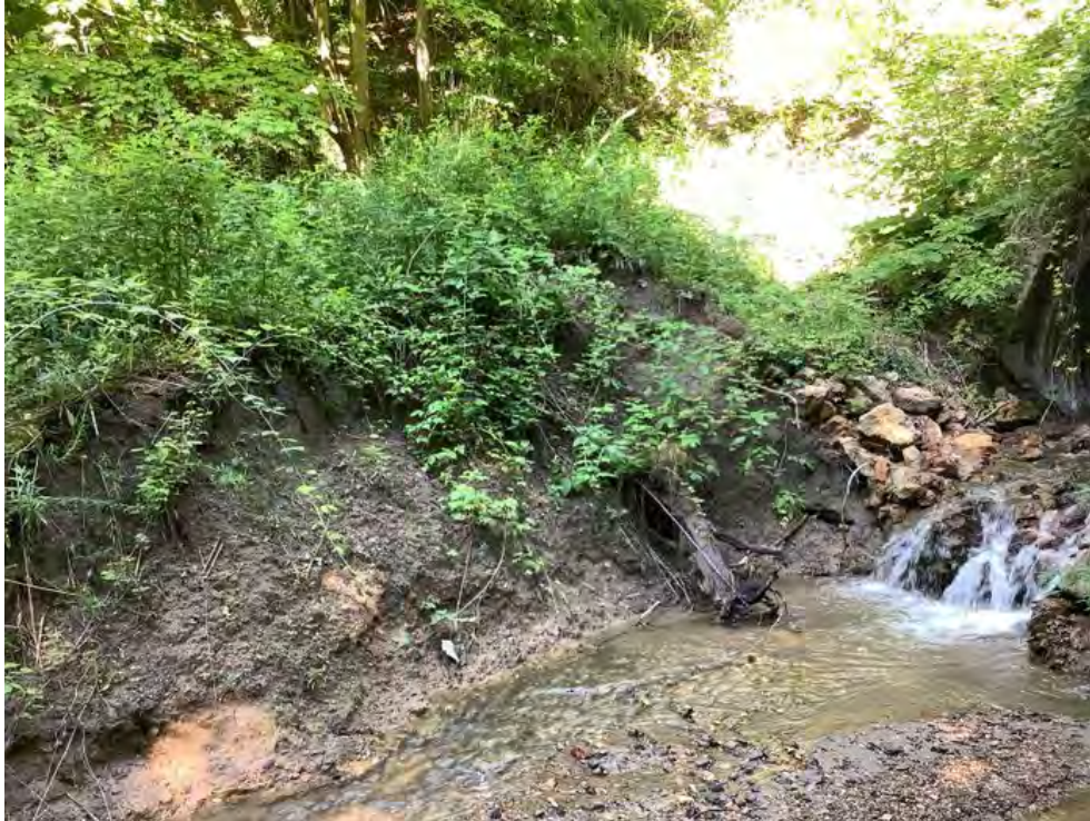
Slumping along the right bank d/s from the outlet
