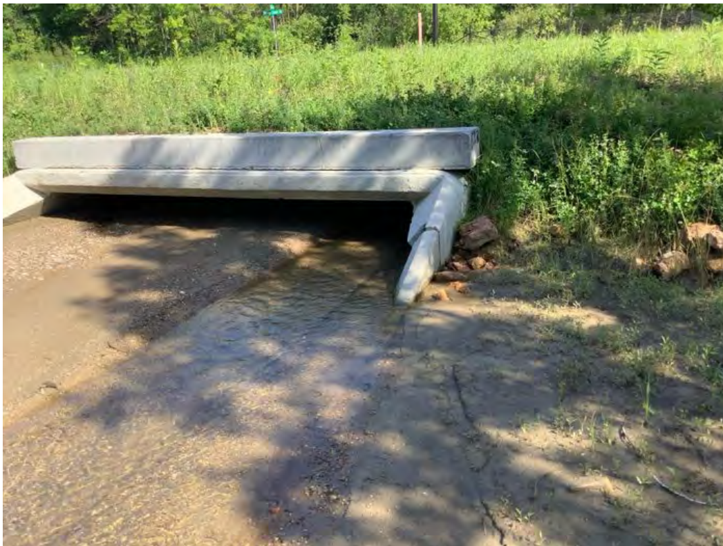
Looking at frontal view of outlet culvert
