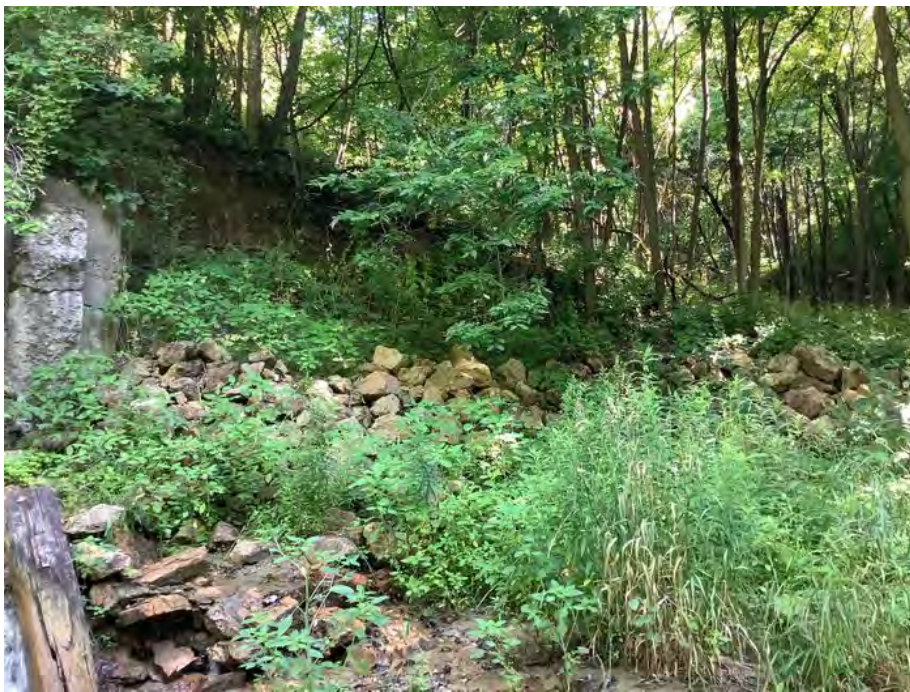
Riprap stabilization along the left bank
