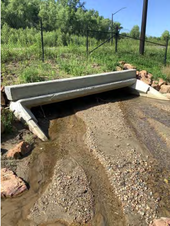
Looking d/s at concrete inlet pipe with riprap along the edges
