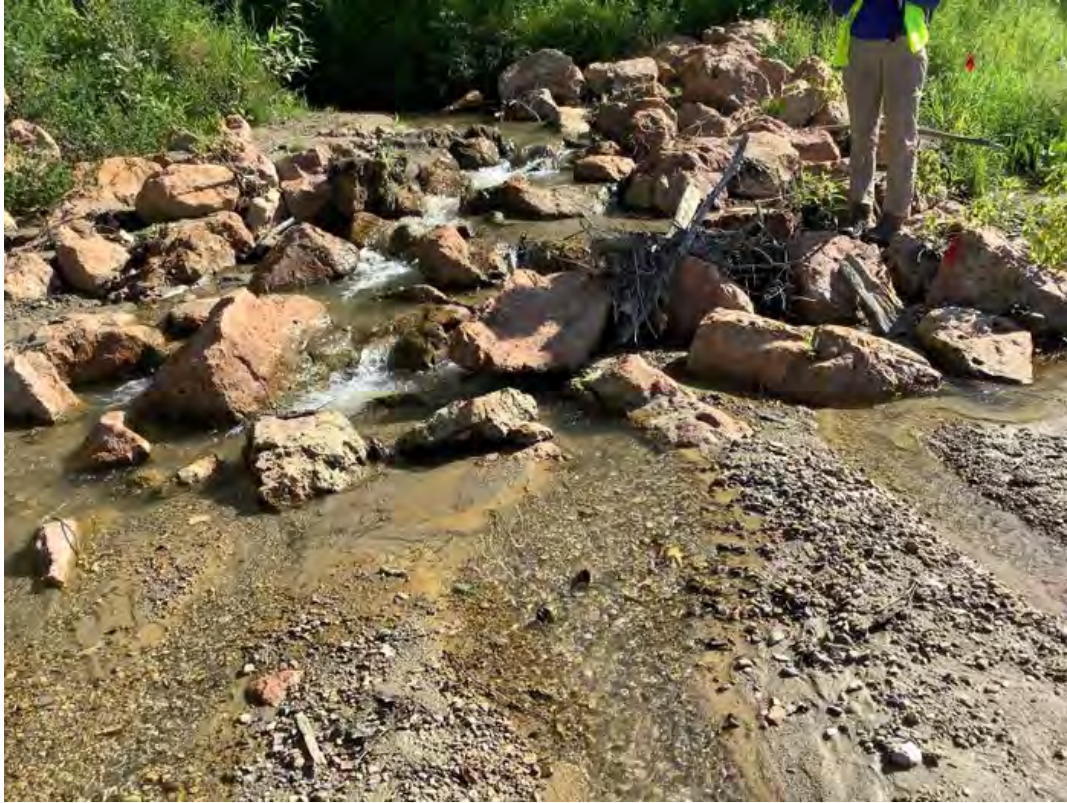
Looking u/s at stream feeding into culvert
