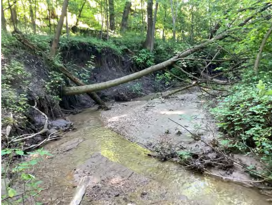
Looking d/s at a large slump with overhang on the left bank
