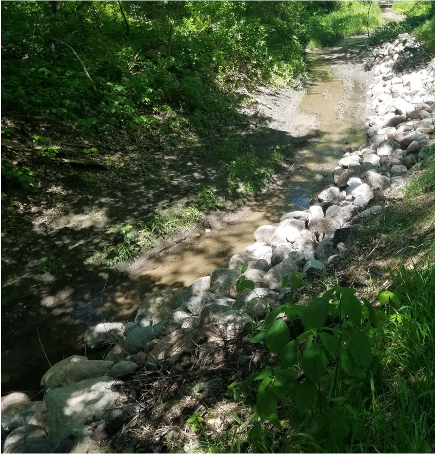
May 28, 2021–Looking upstream from cross-vane structure at left bank toe protection.
