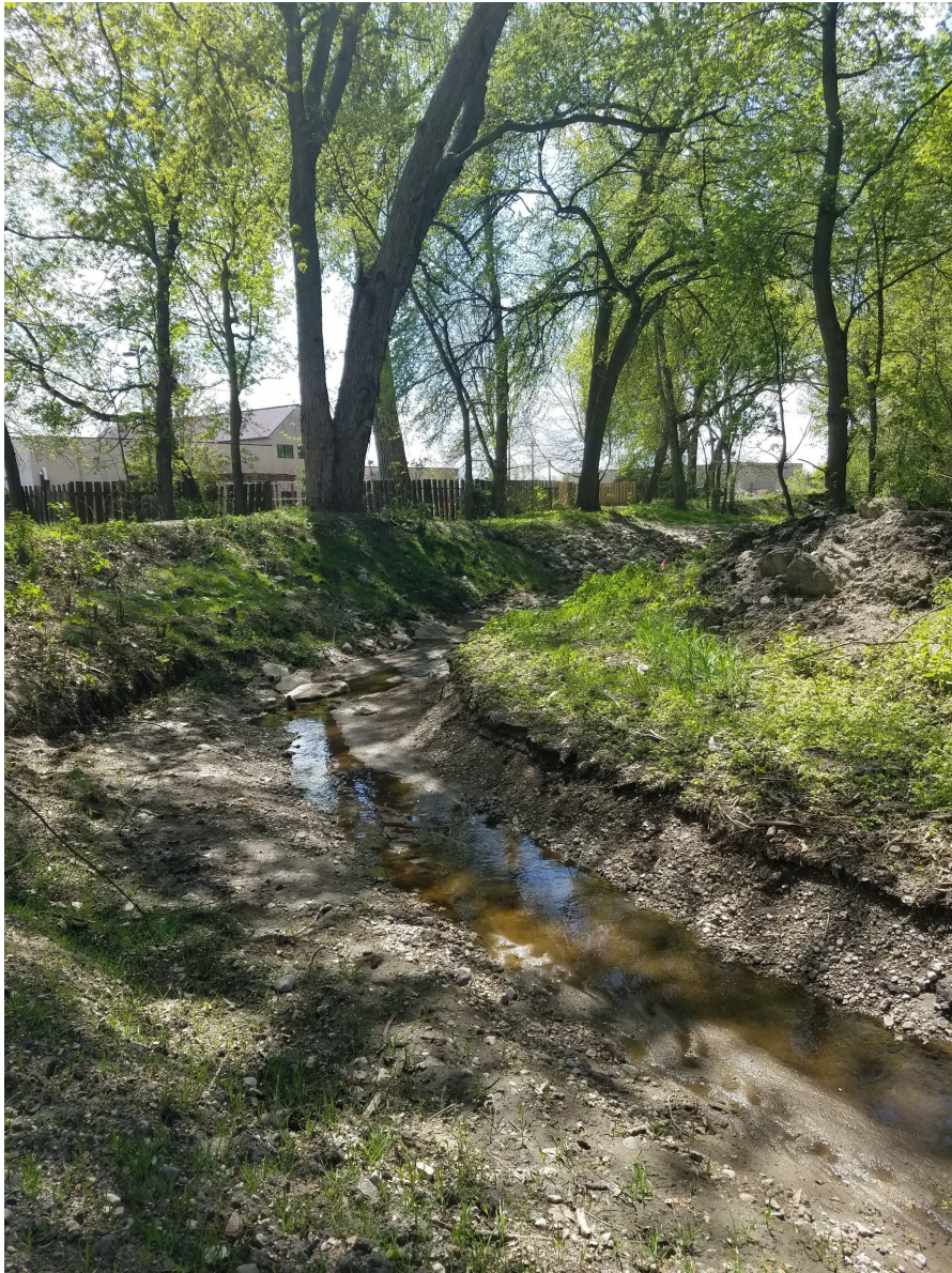
May 6, 2021—Looking downstream at right bank spoils pile before final grading.
