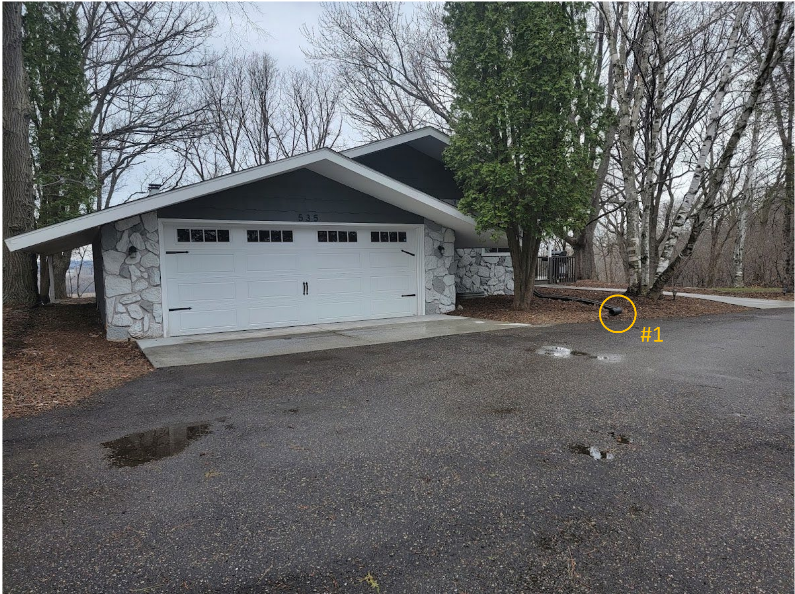
535 Lakota Lane – front of house (discharge points circled in yellow)
