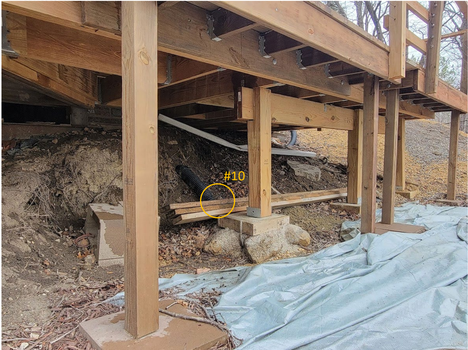
535 Lakota Lane – south side of house, under new deck
