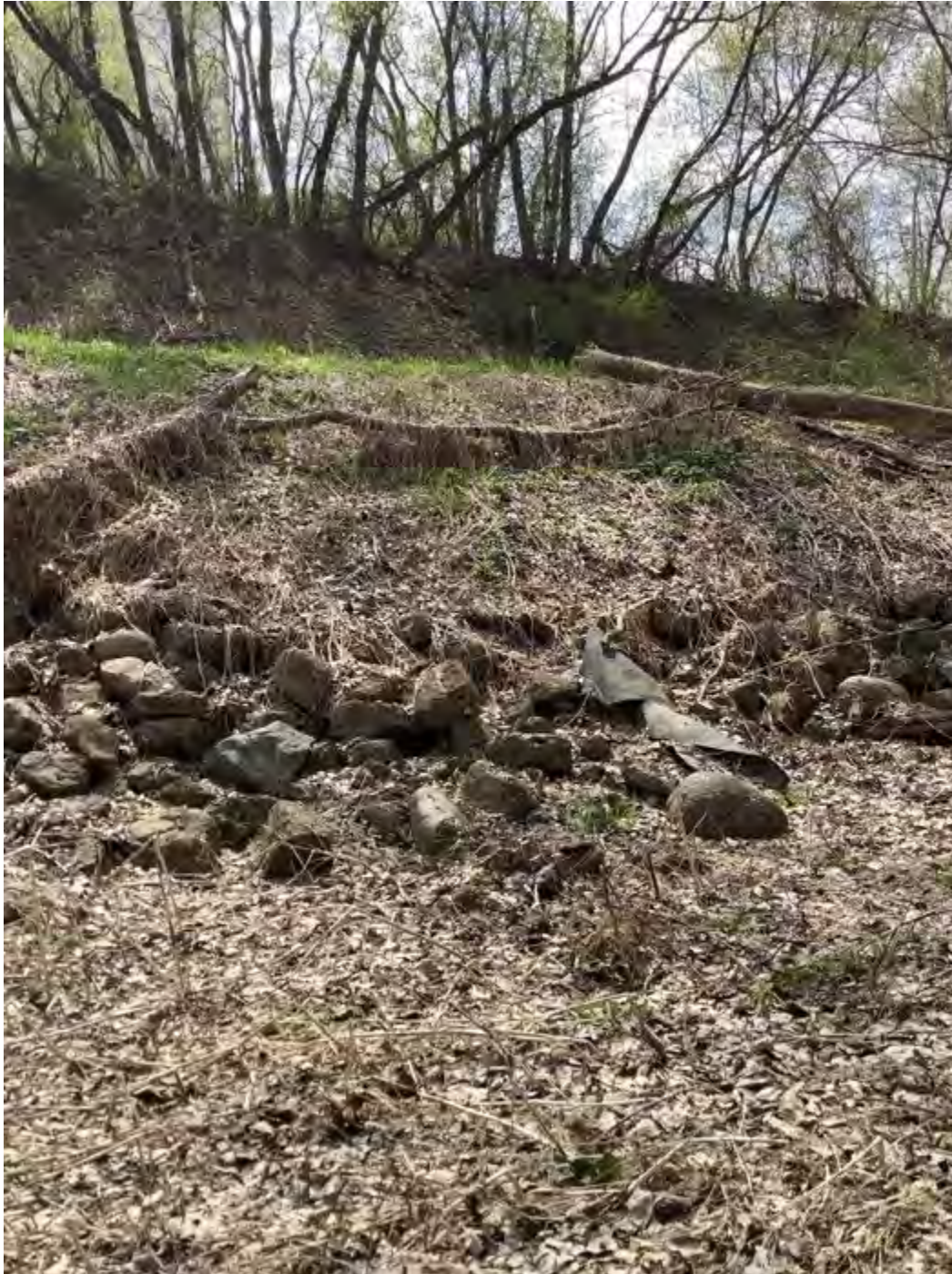
Bank reinforcing stones
