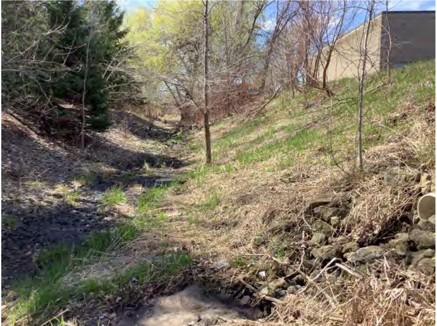
Top of gully
