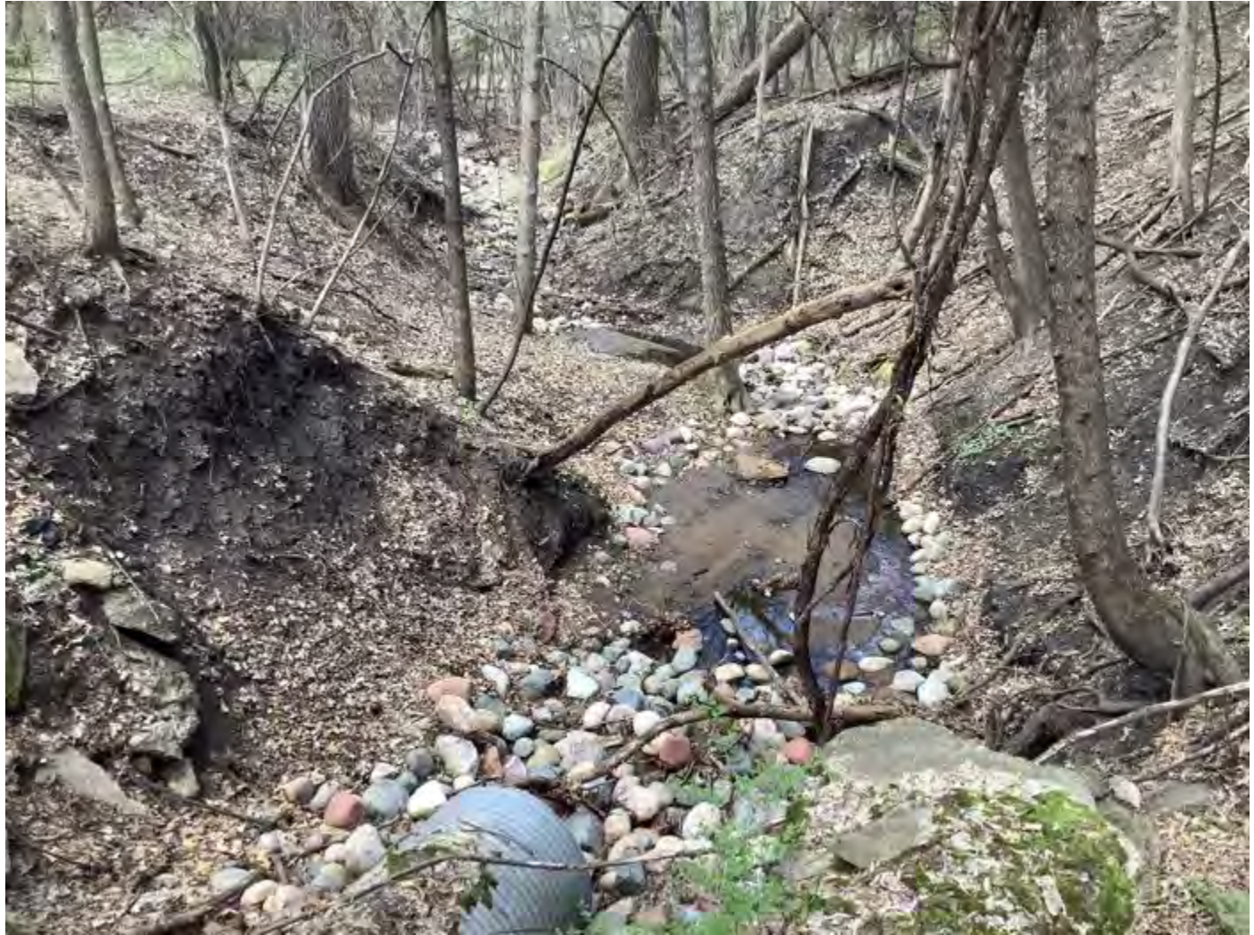
150ft down trail
