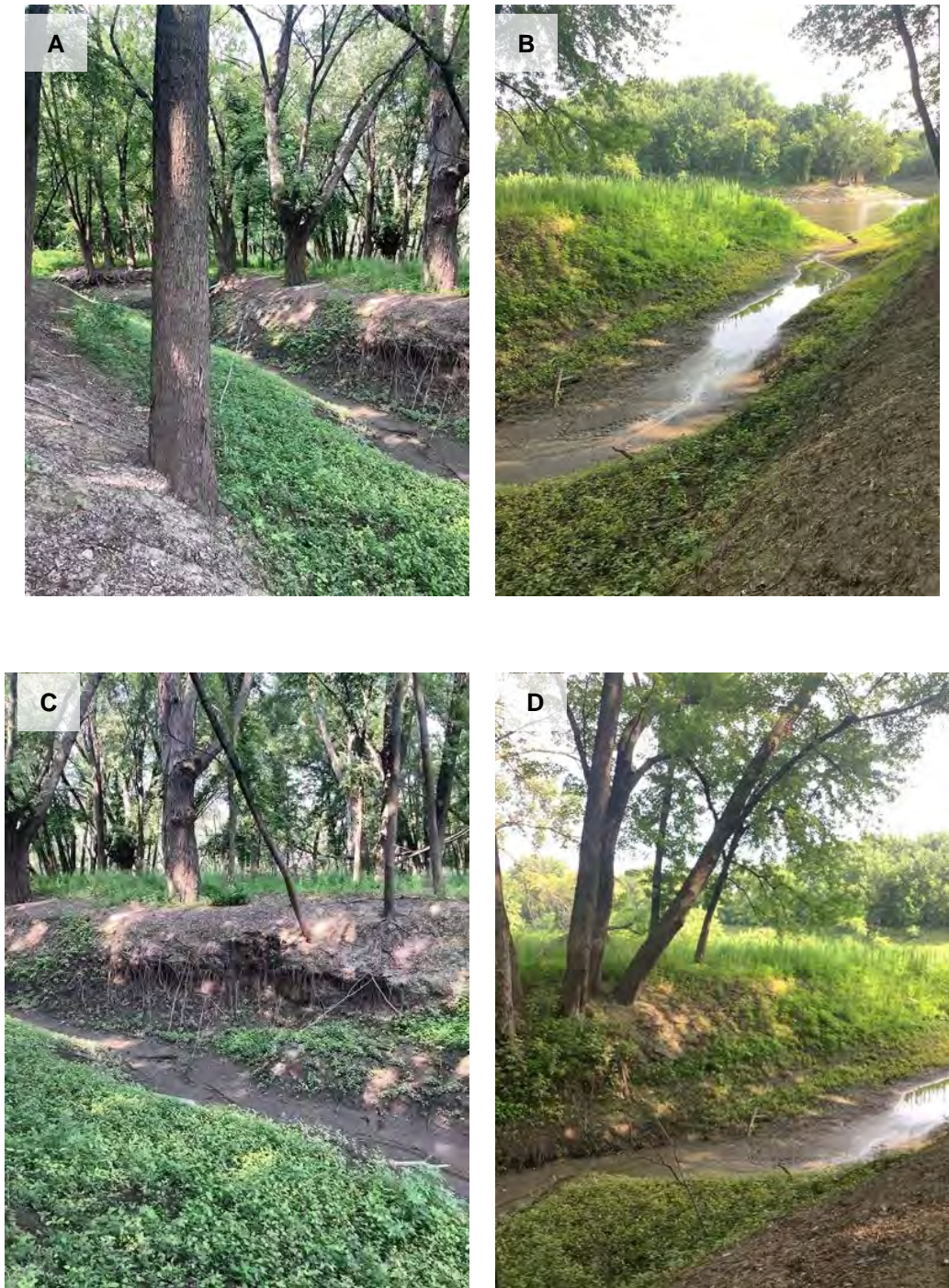
Figure 32: Photos of Gully 07:12-10:13. A) Upstream view of gully, B) Downstream view of confluence with Minnesota River, C) View of severe degradation on left bank, D) View of leaning trees on right bank
