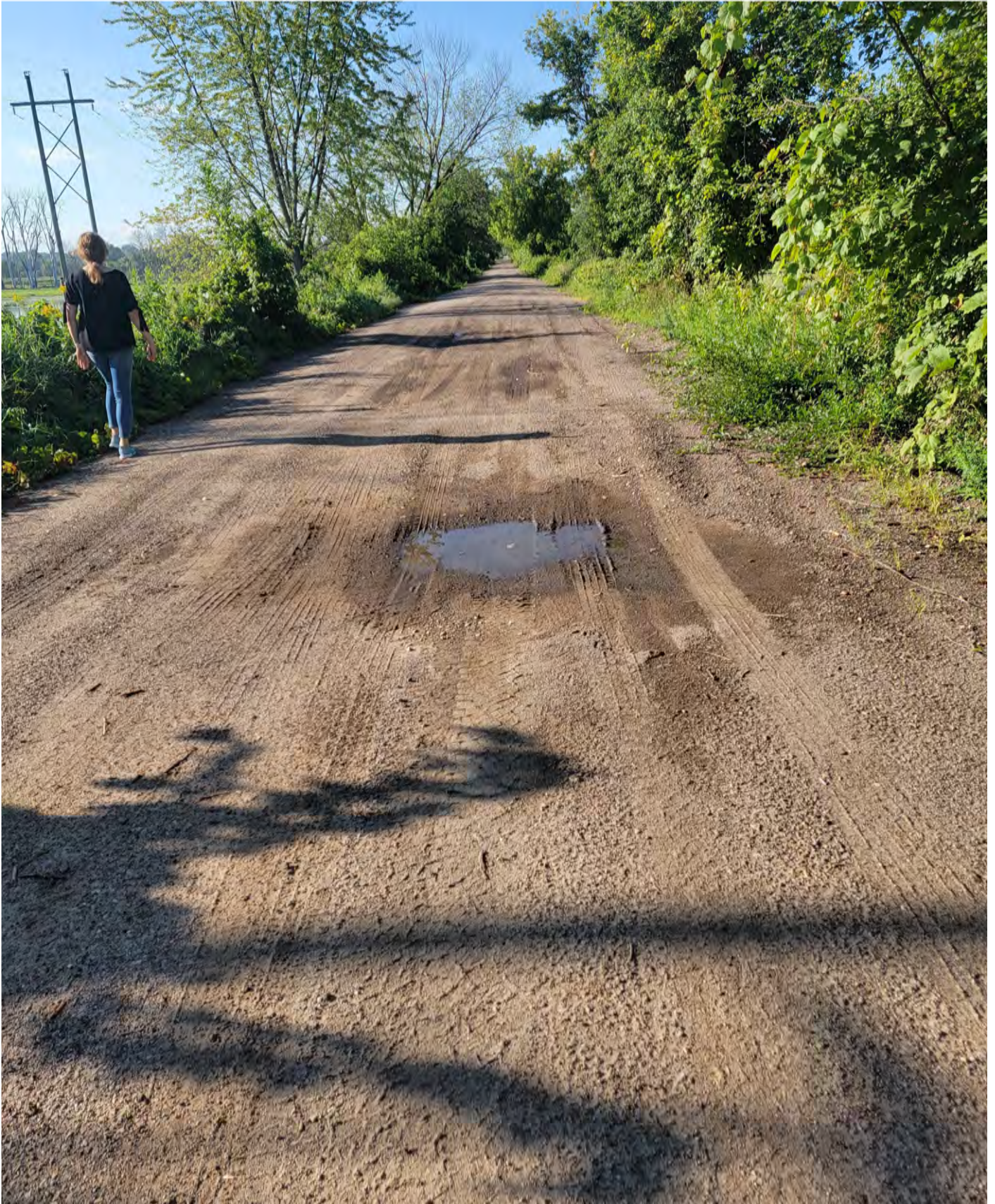
Photo 3A. Vernon Avenue looking south. In 2015, the AET soil boring B-3 indicated the roadway was reduced to 0.25-inch chip seal layer atop 11.5-inches of sandy fill.
