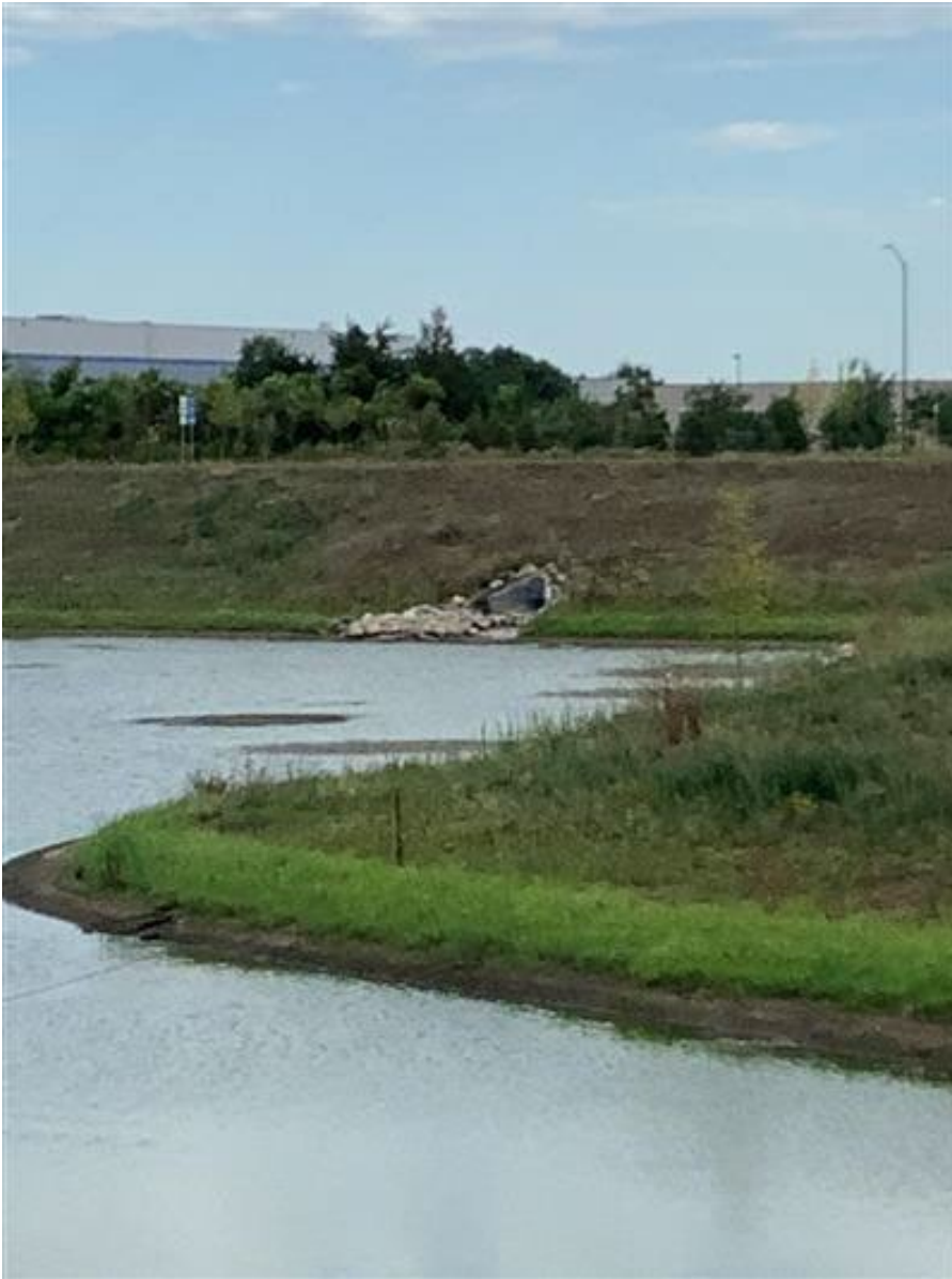
Figure 2. Culvert in northwest regional pond
