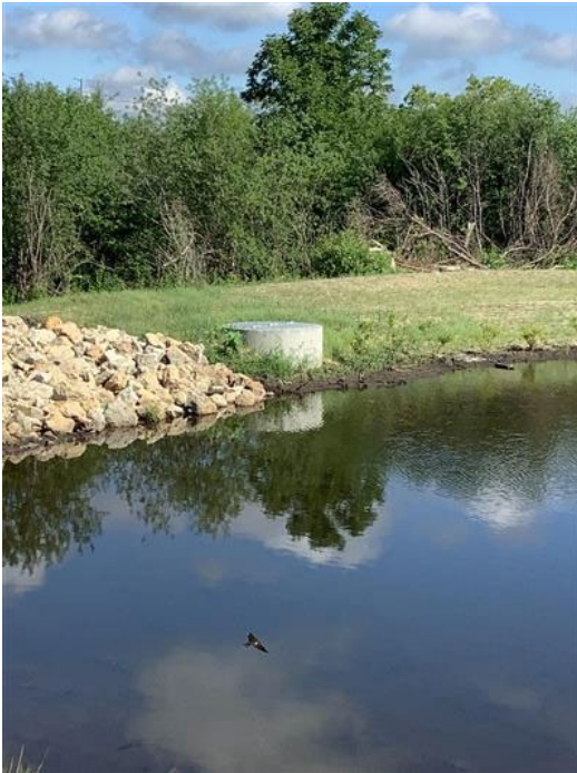
Figure 3. Western emergency overflow
