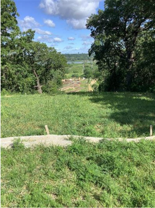
Figure 3 - South slope breakers at the top of hill
