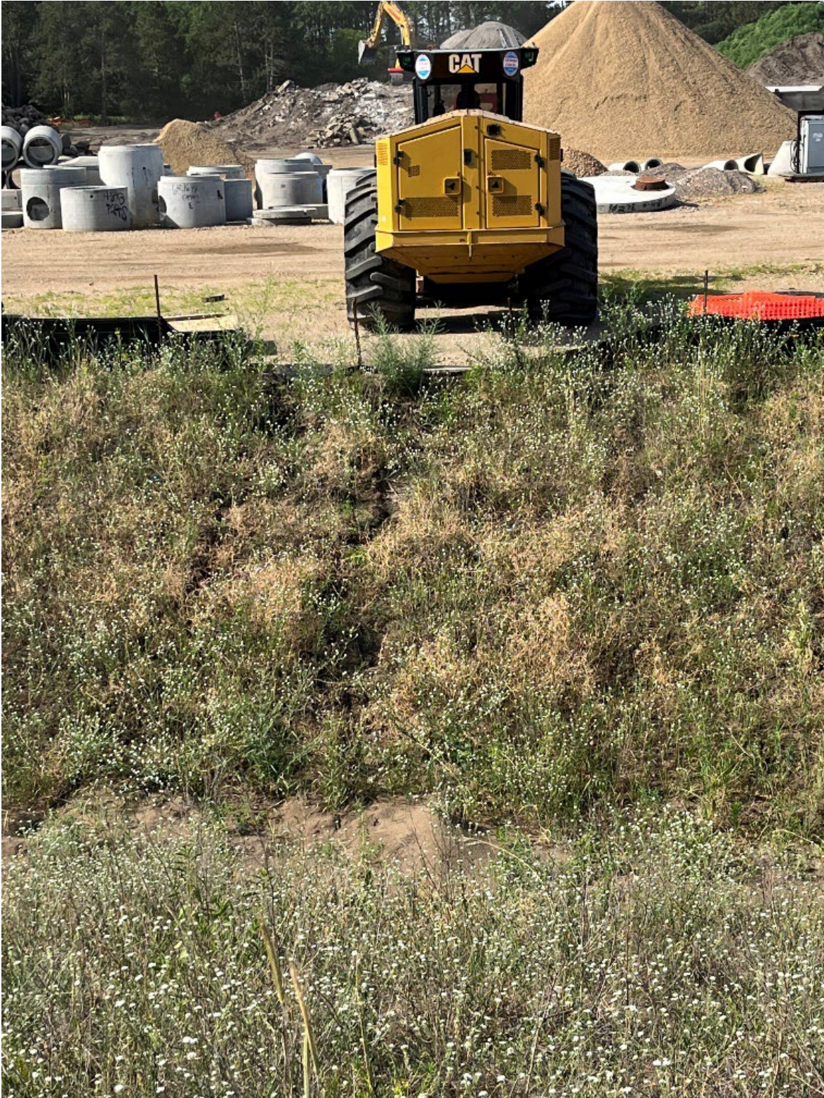
Figure 2. Rill formation in pond sidewall
