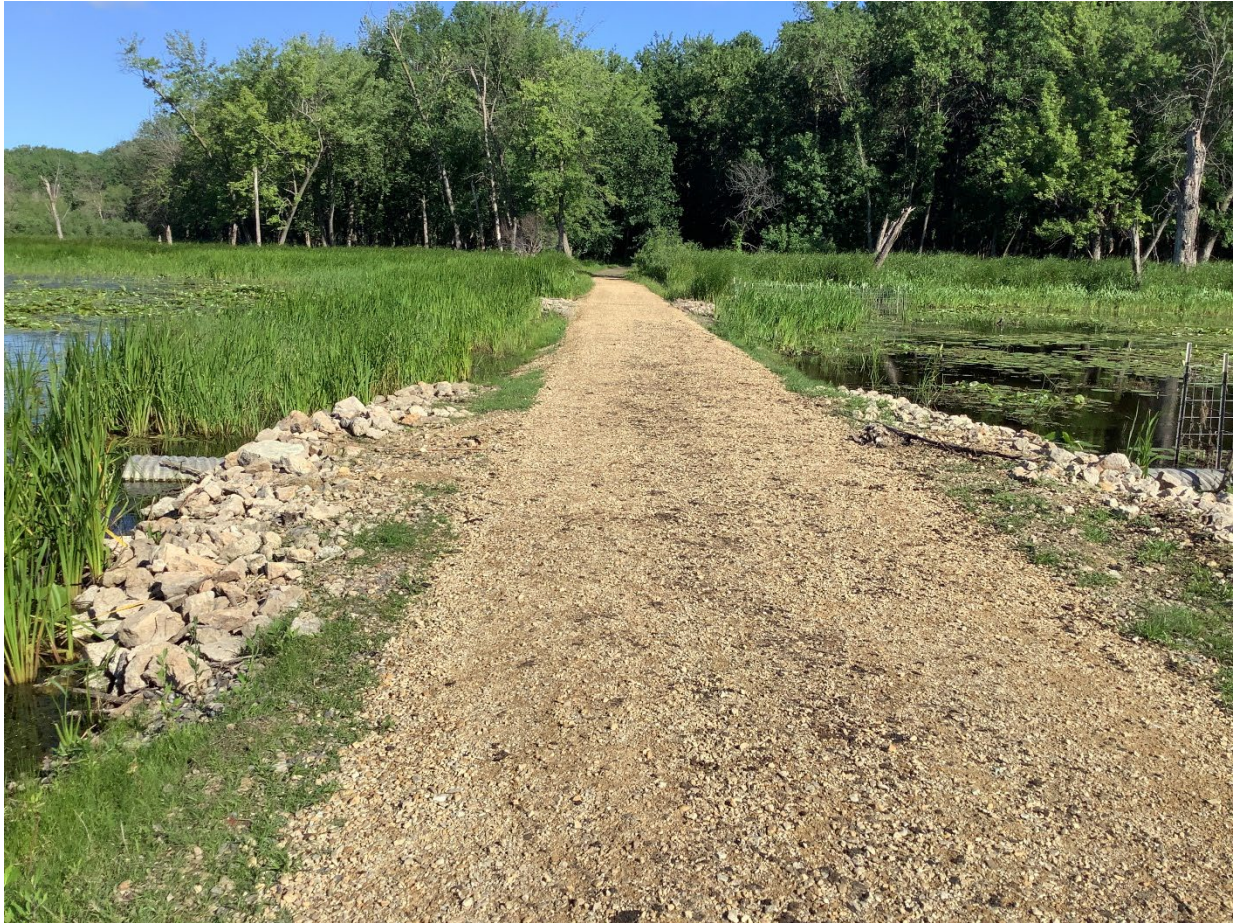
Figure 1. South culvert replacement area
