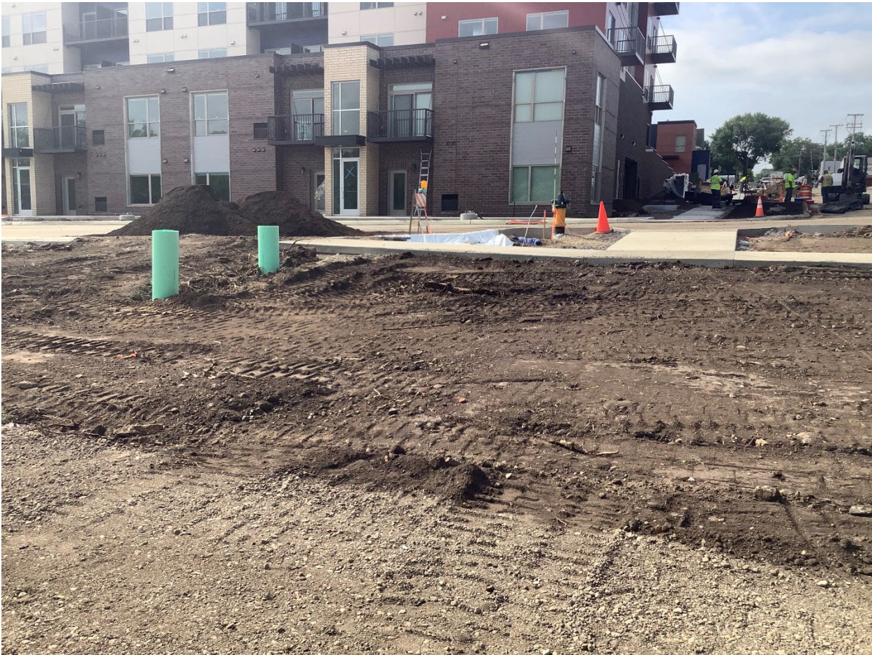
Figure 3. Underground stormwater management facility under construction
