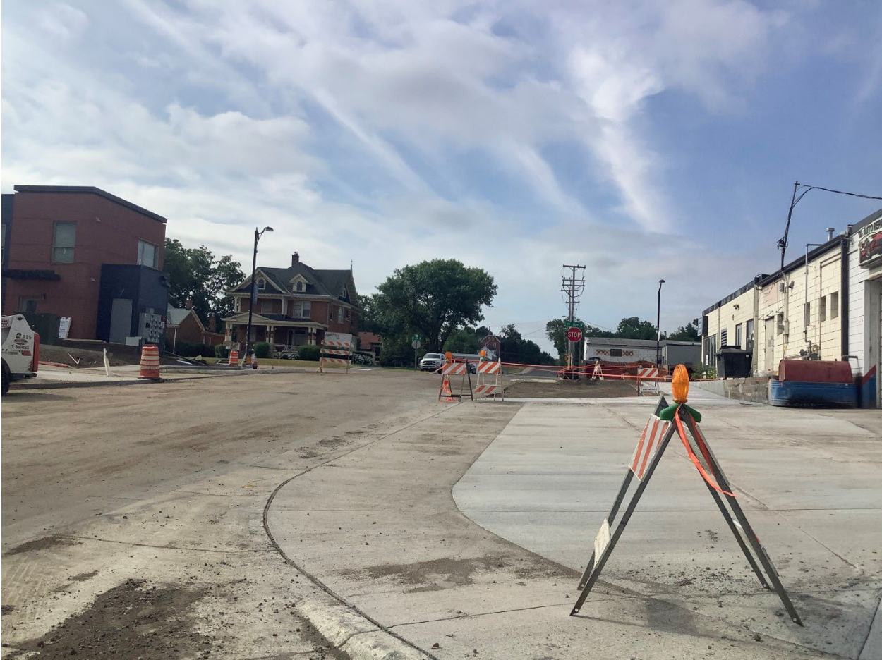
Figure 3. Current construction on Scott St
