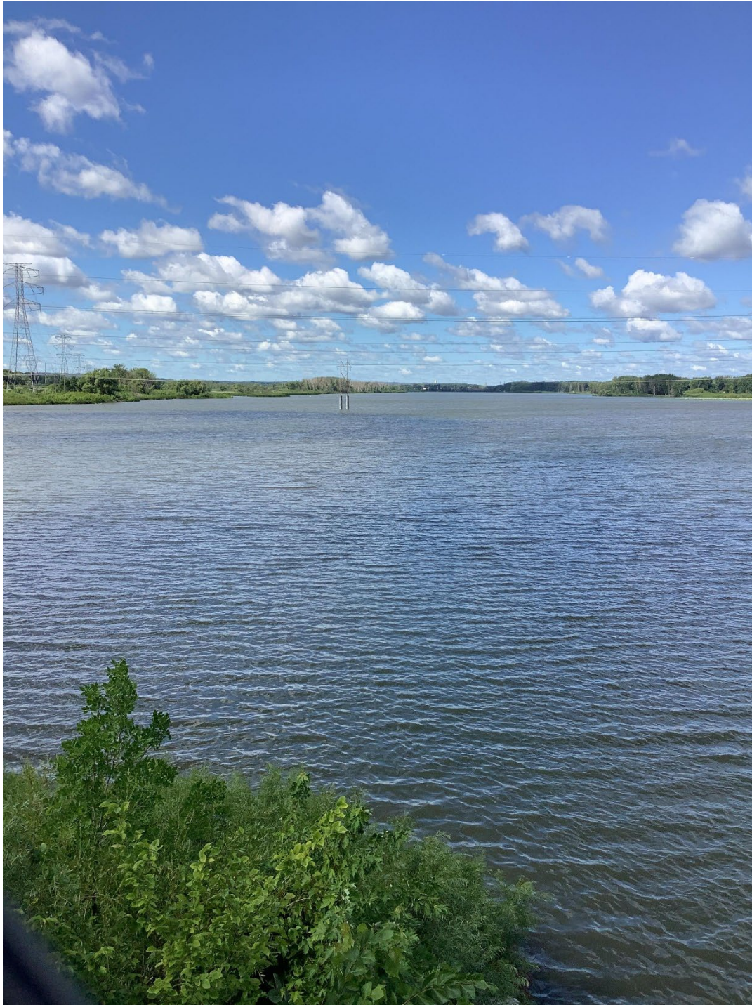
Figure 1. Repaired line in Black Dog Lake
