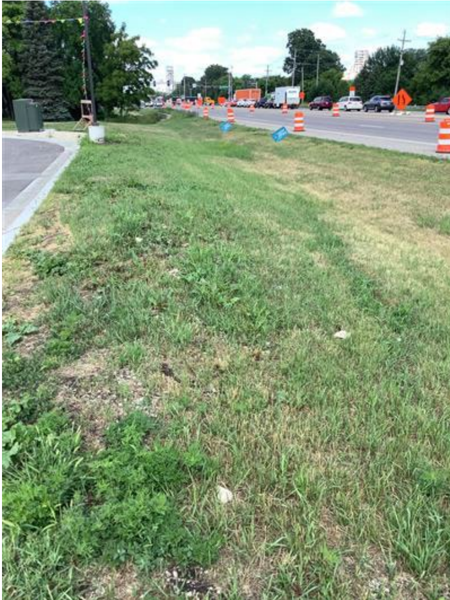
Figure 1. Greater than 70 percent vegetative stabilization on site
