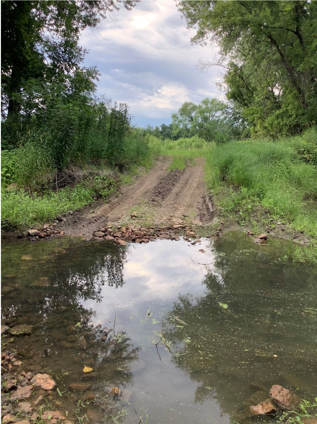
Figure 1. Road entrance with dip looking south
