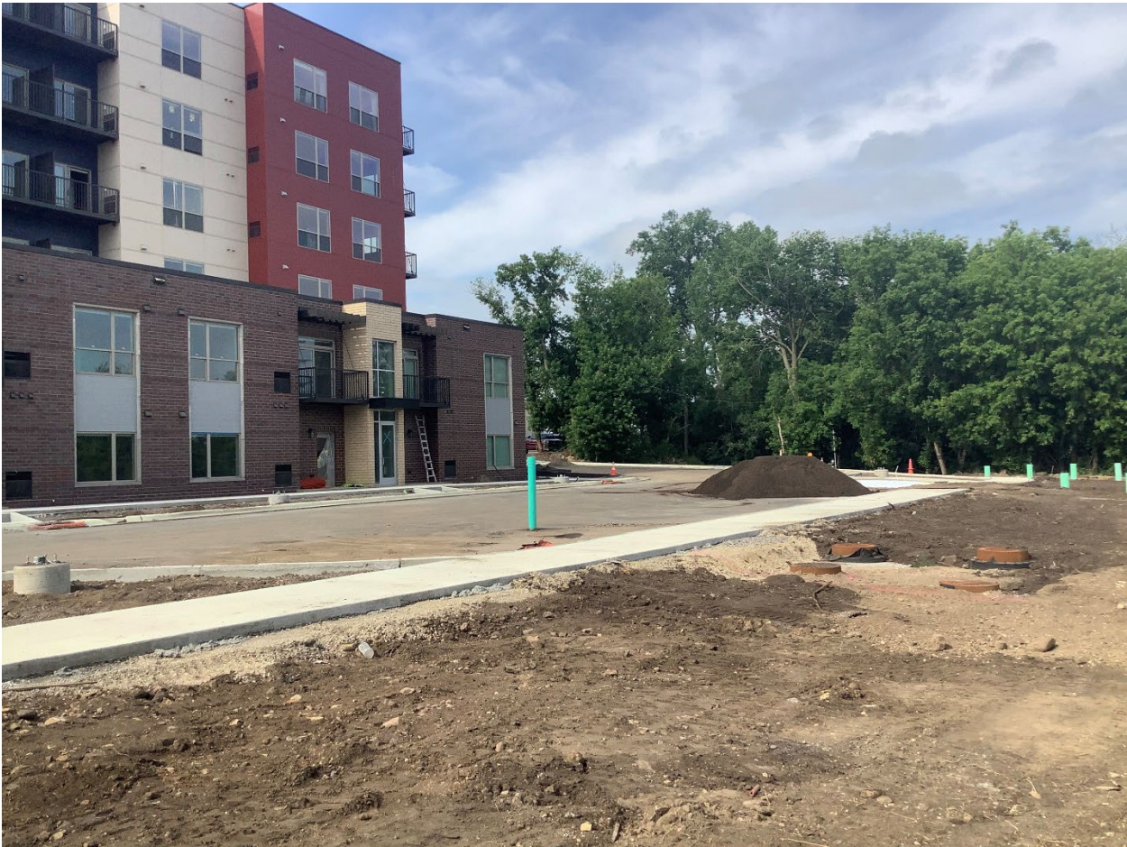
Figure 2. Parking lot and building on Levee Drive
