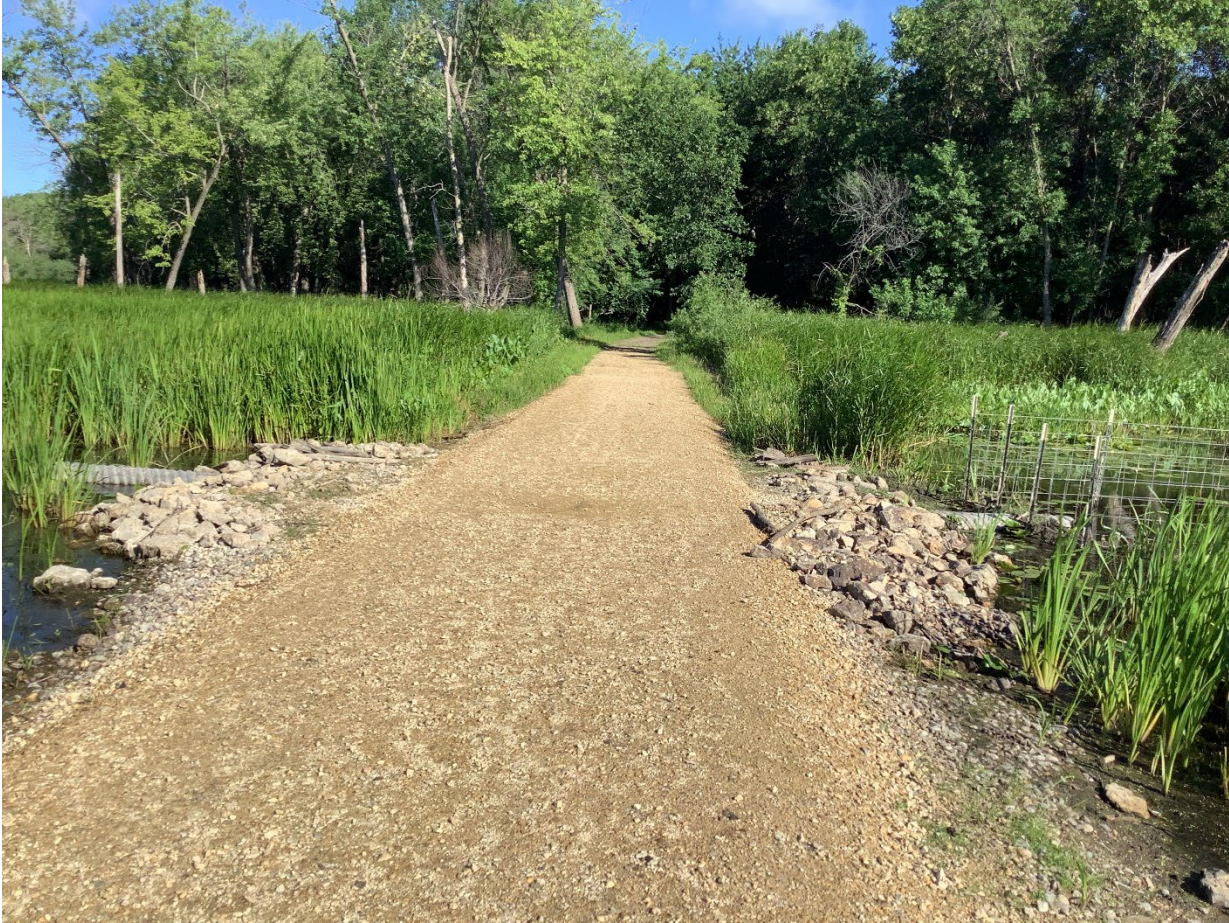
Figure 2. North culvert replacement area
