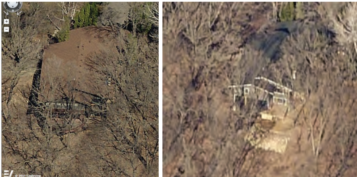
Figure 3. Carver County aerial images of 535 Lakota Lane (left taken April 15, 2015, and right taken November 21, 2020.).
