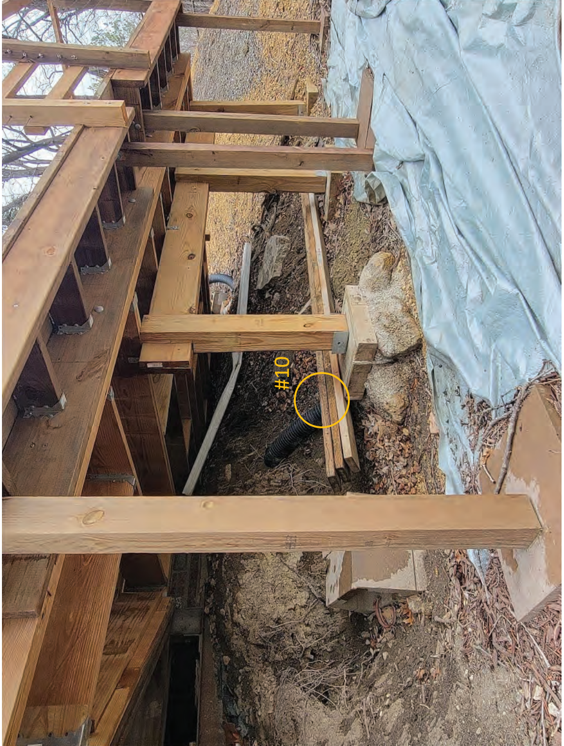
535 Lakota Lane – south side of house, under new deck
