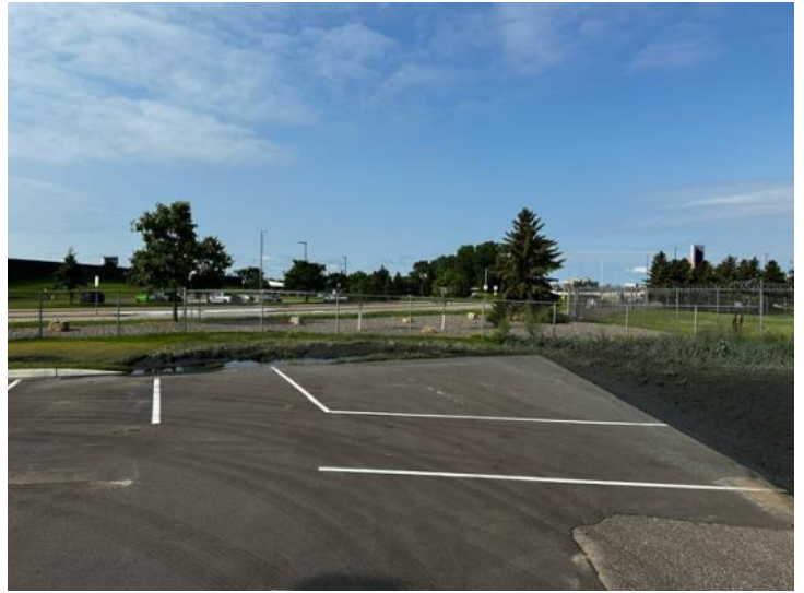
Photo 4 Correction - Hydroseeding on west side of project
