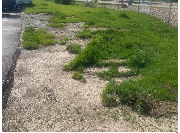
Photo 2 Violation - Exposed soils on west side of project site
