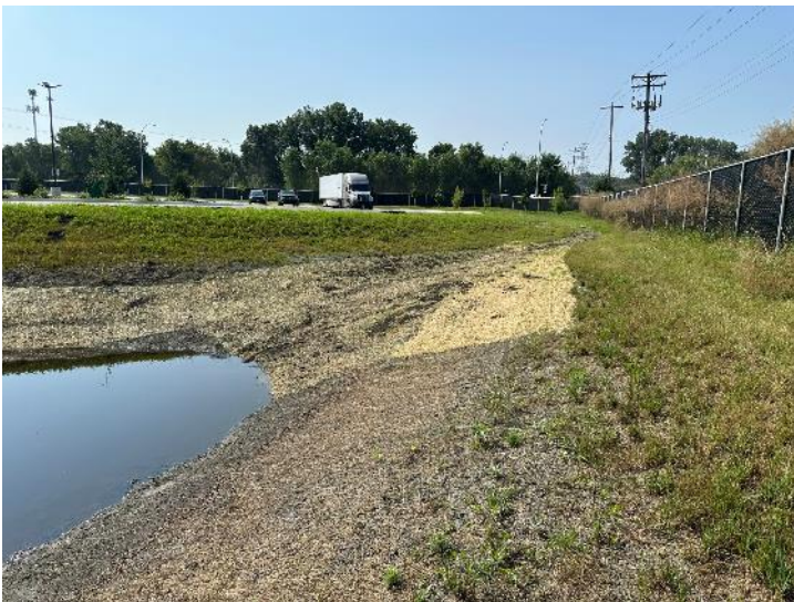
Photo 5 Correction - Erosion control blanket applied to southwest corner of pond
