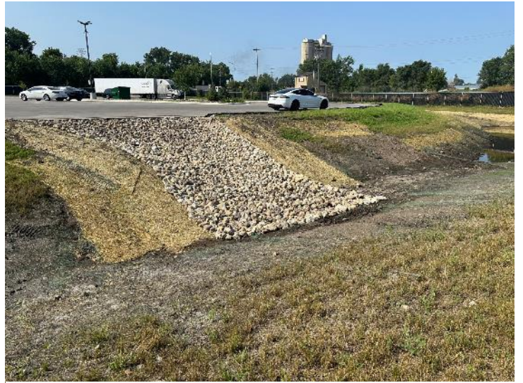
Photo 4 Correction - Rip rap channel widened and erosion control blanket applied
