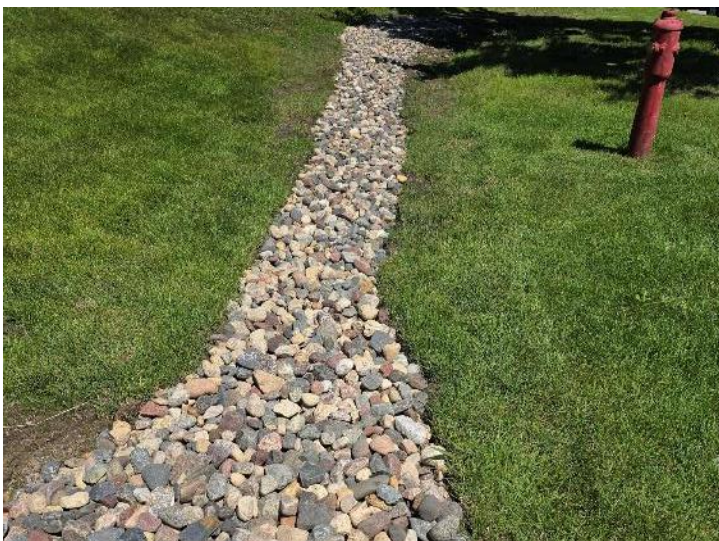
Photo 5 Correction - Rock drainage (dry creek) installed
