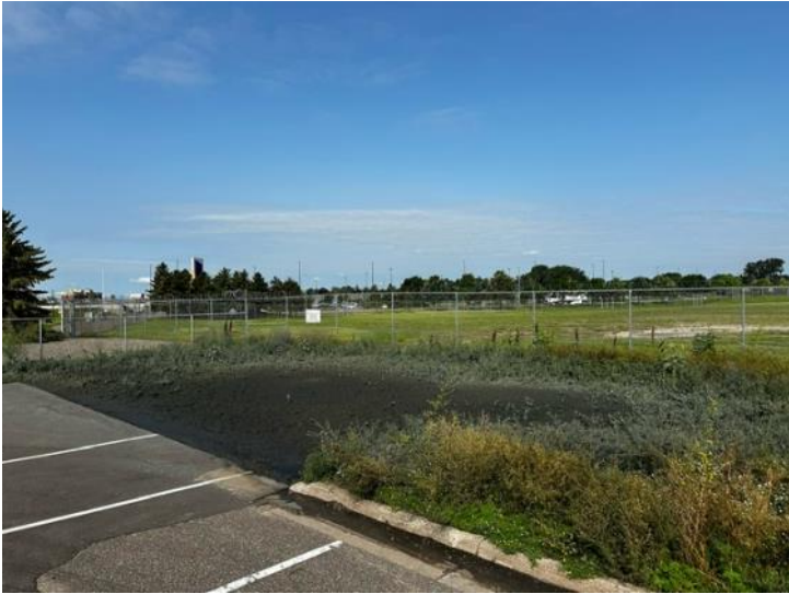
Photo 3 Correction - Hydroseeding on west side of project
