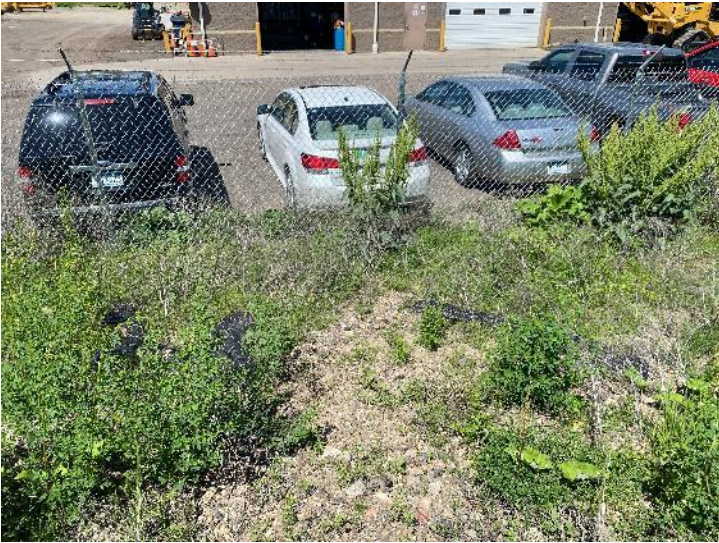
Photo 3 Violation - Temporary BMPs and hillslope erosion
