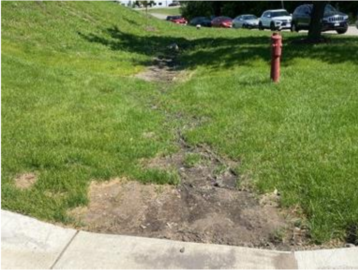
Photo 1 Violation - Erosion and exposed soils from curb cut to catch basin.
