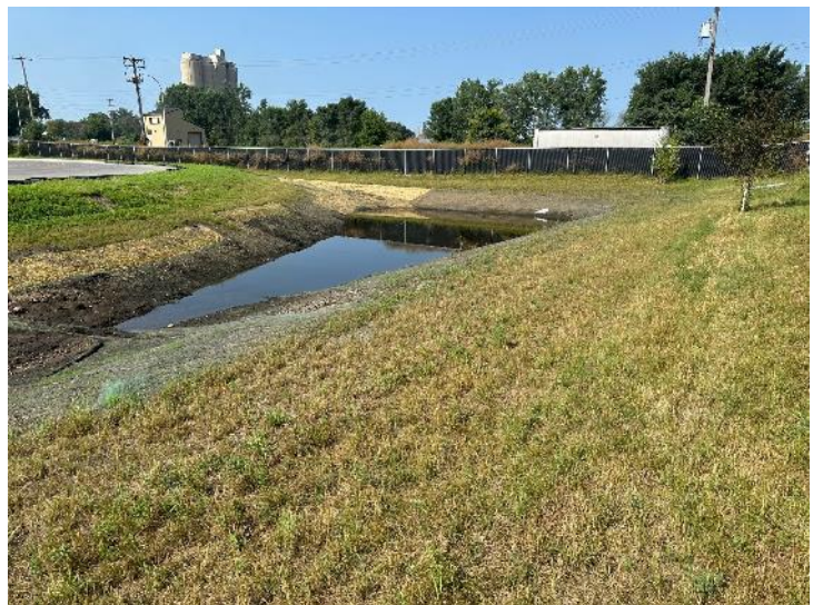
Photo 6 Correction - Erosion control blanket applied
