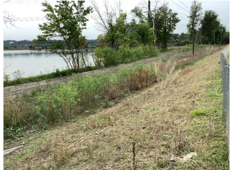
Figure 2: <70% Vegetation Establishment at I35W Frontage Trail
