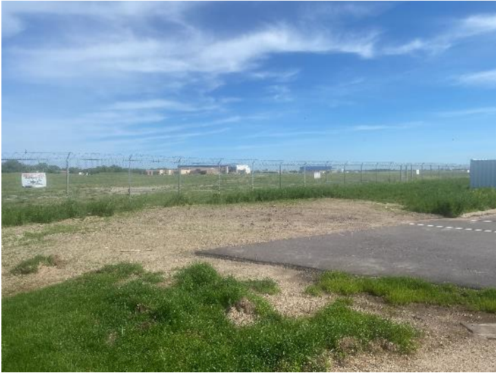
Photo 1 Violation - Exposed soils on west side of project site
