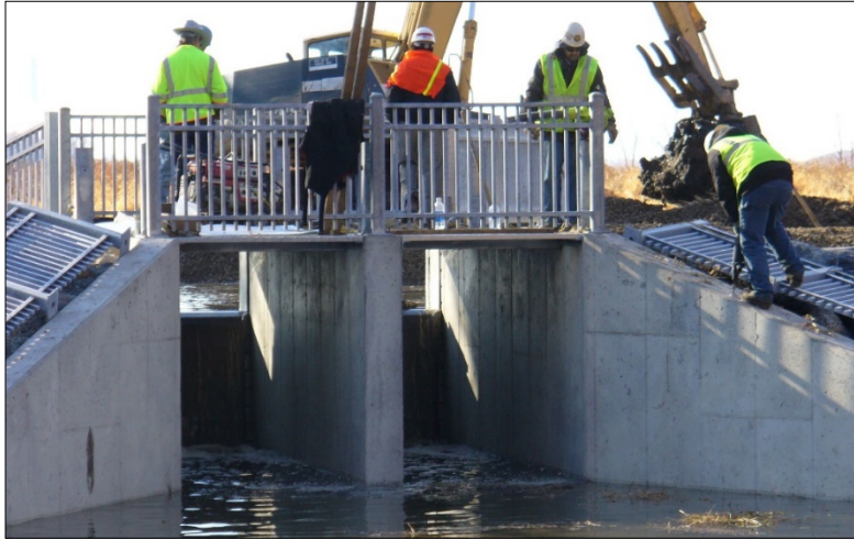
Figure 2: Long Meadow Lake water control structure during handrail construction
