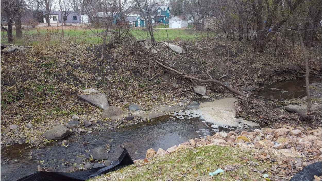
Photo 7: Site M10 – debris in channel downstream of site repaired by city of Chaska
