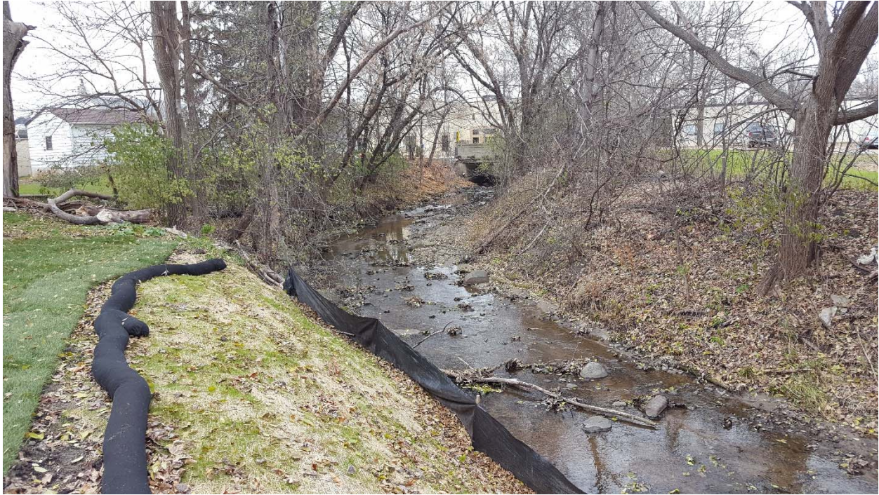
Photo 17: Site S7 – recent repairs made by city of Chaska
