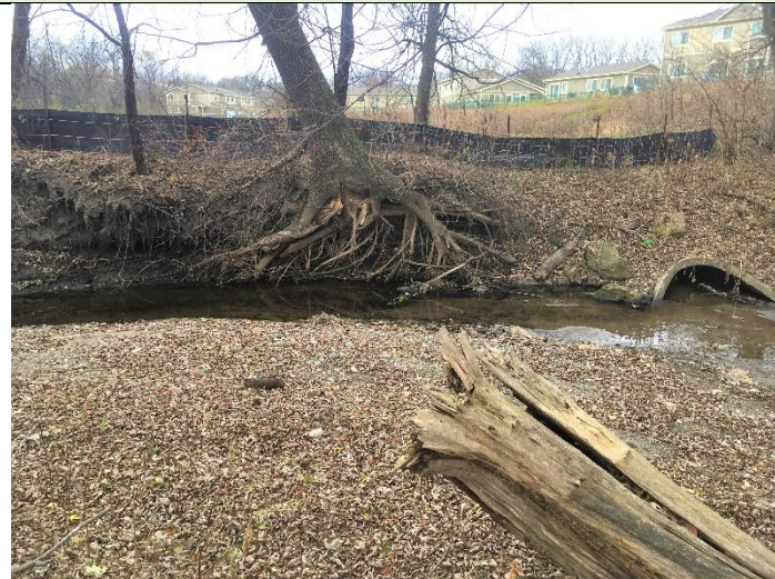
Nov. 2018 Field Visit: Eroded bank slightly upstream for dual outfalls.
