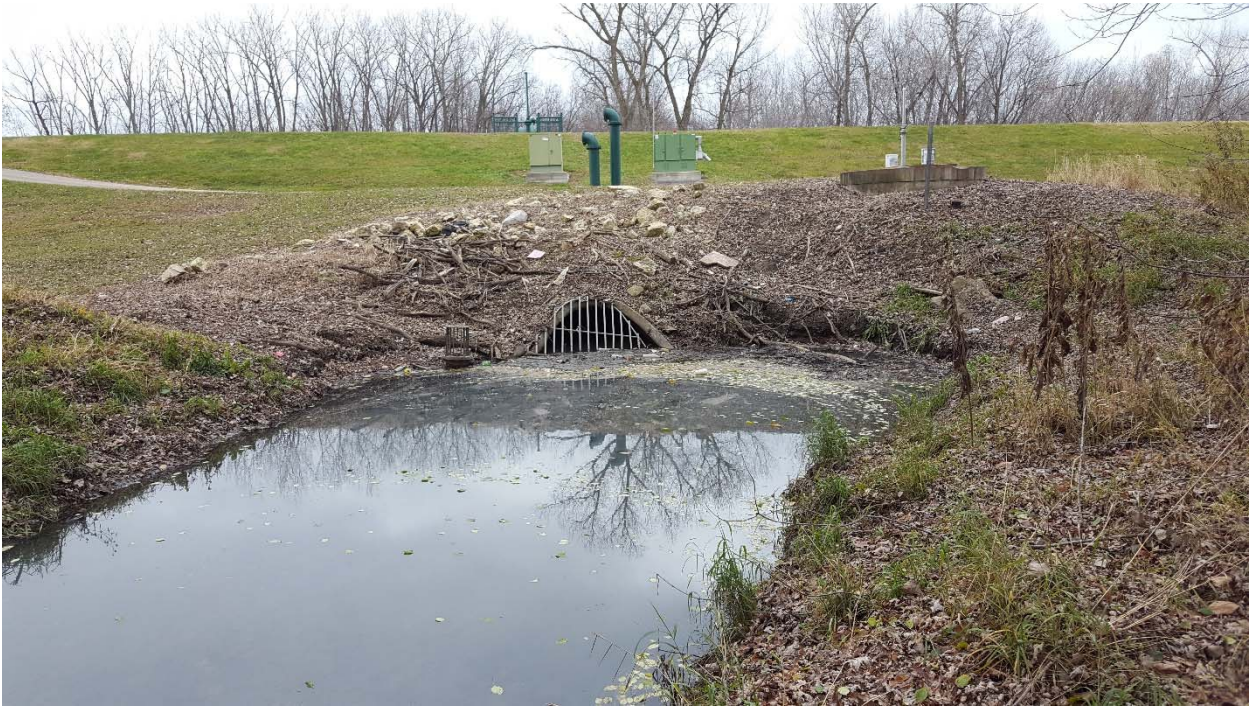
Photo 10: Site M13 – culvert outlet through the levee.
