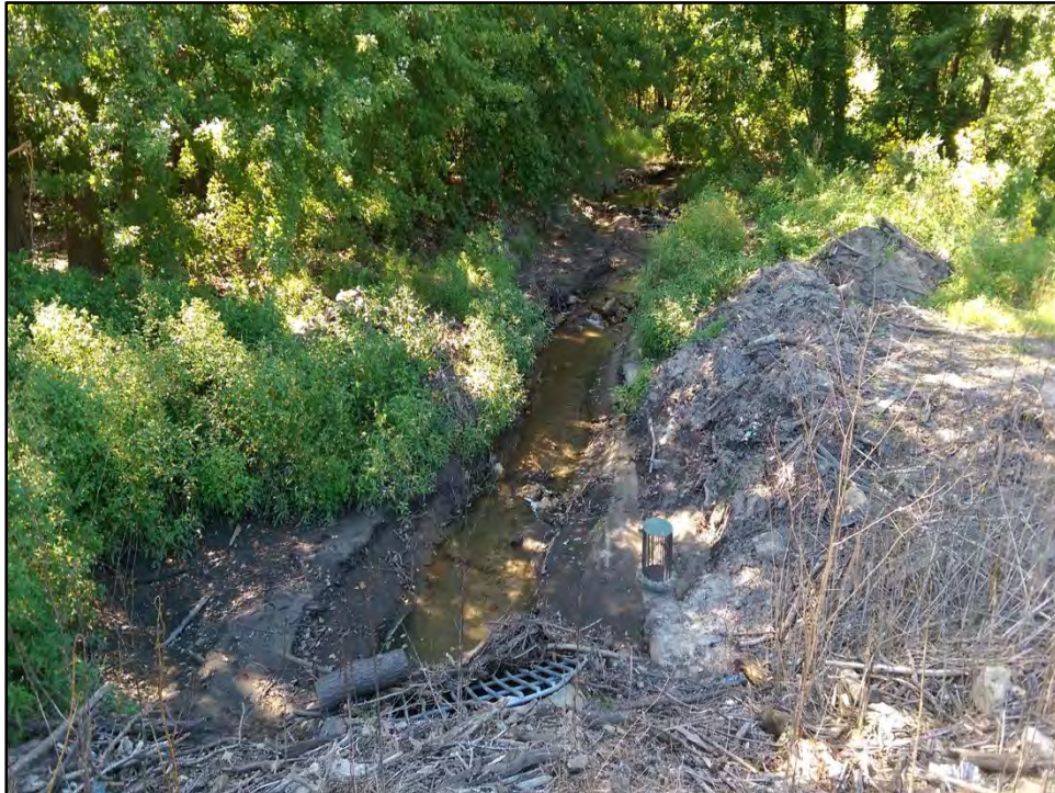
Photograph C-5: View south of debris and potential settling basin.
