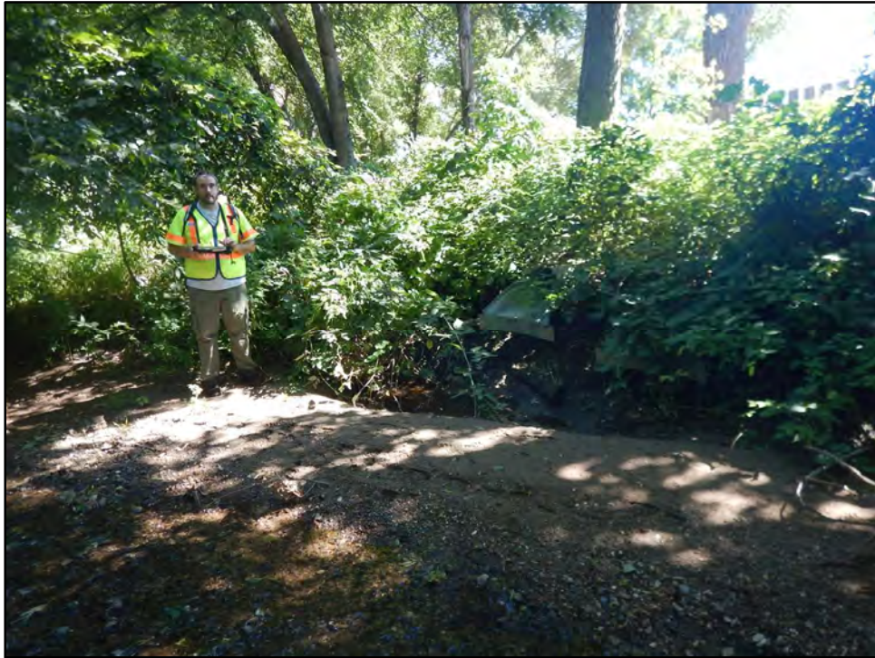
Photograph A-2: View east of dual 12" CMP outfalls.
