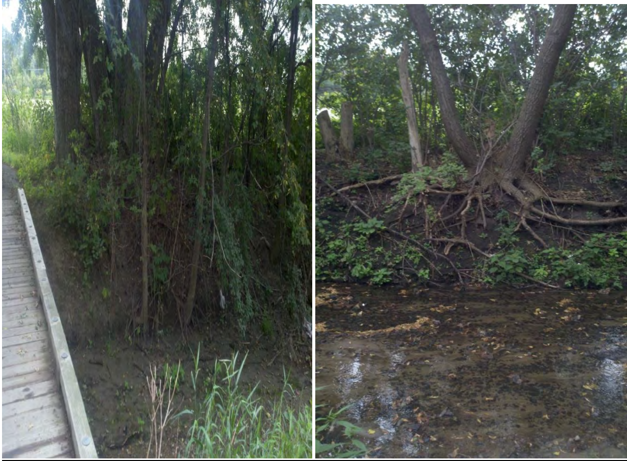
Photo 11. Pedestrian bridge north of CR 61 and downstream, East Chaska Creek
