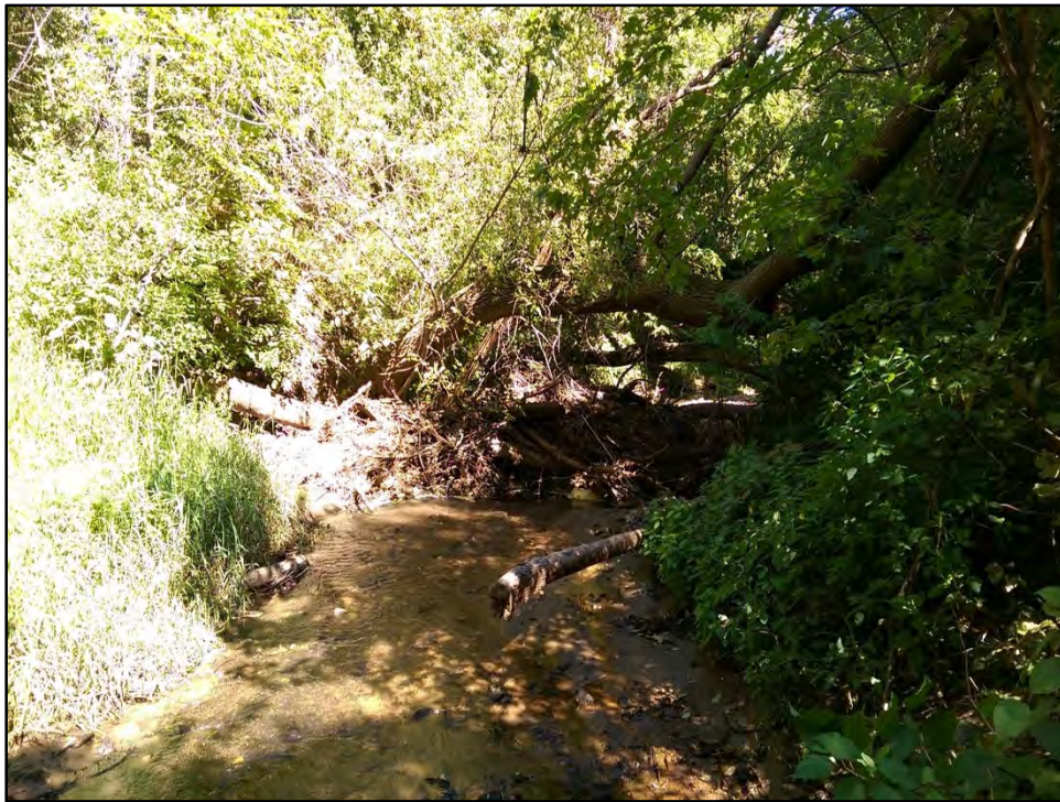
Photograph A-13: View east of debris.
