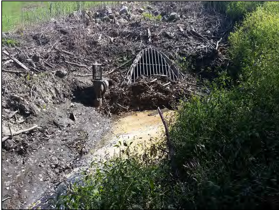
Photograph C-6: View east of debris, creek levee crossing, and potential settling basin.
