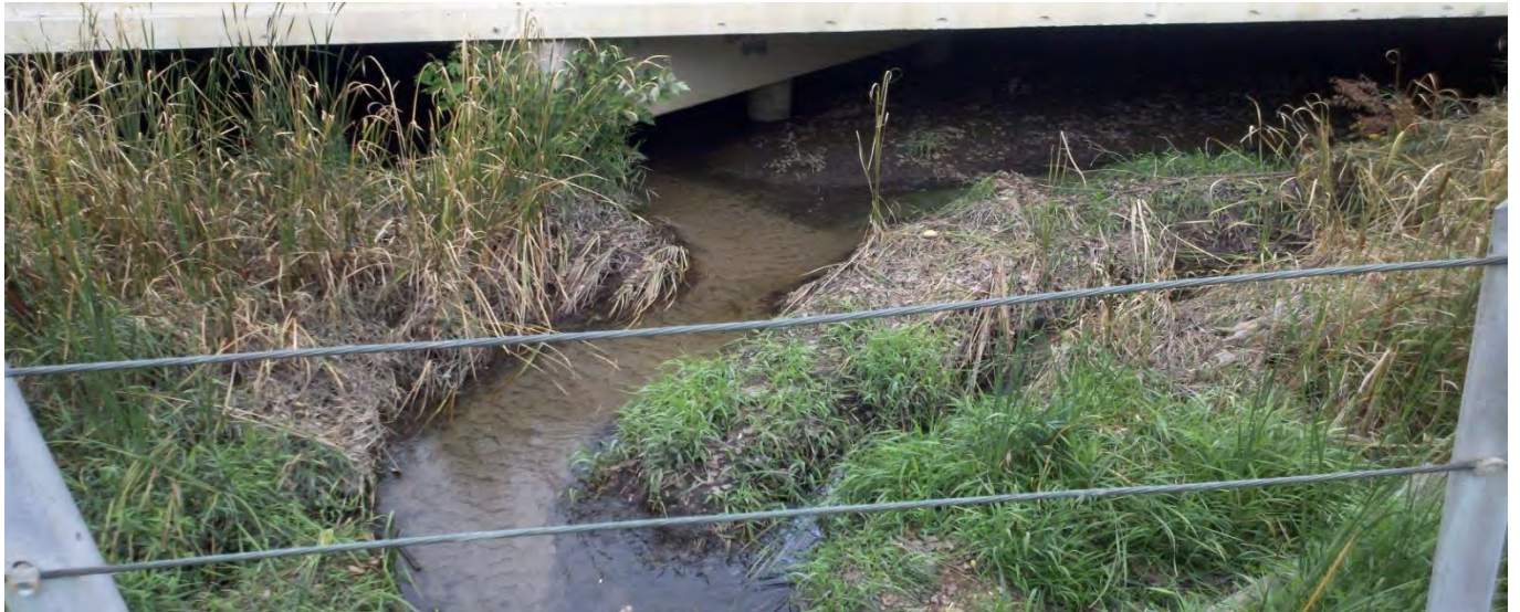
Photo 13. Downstream of County Road 61, East Chaska Creek
