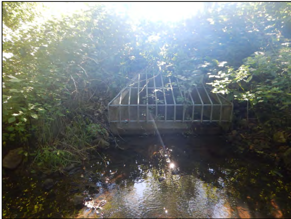
Photograph A-1: View east of RCP outfall.
