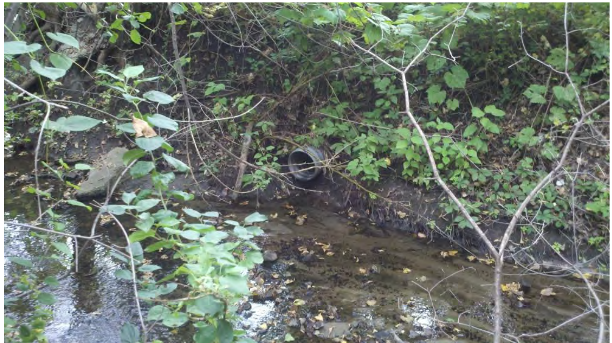
Photo 10. Outfall C, East Chaska Creek
