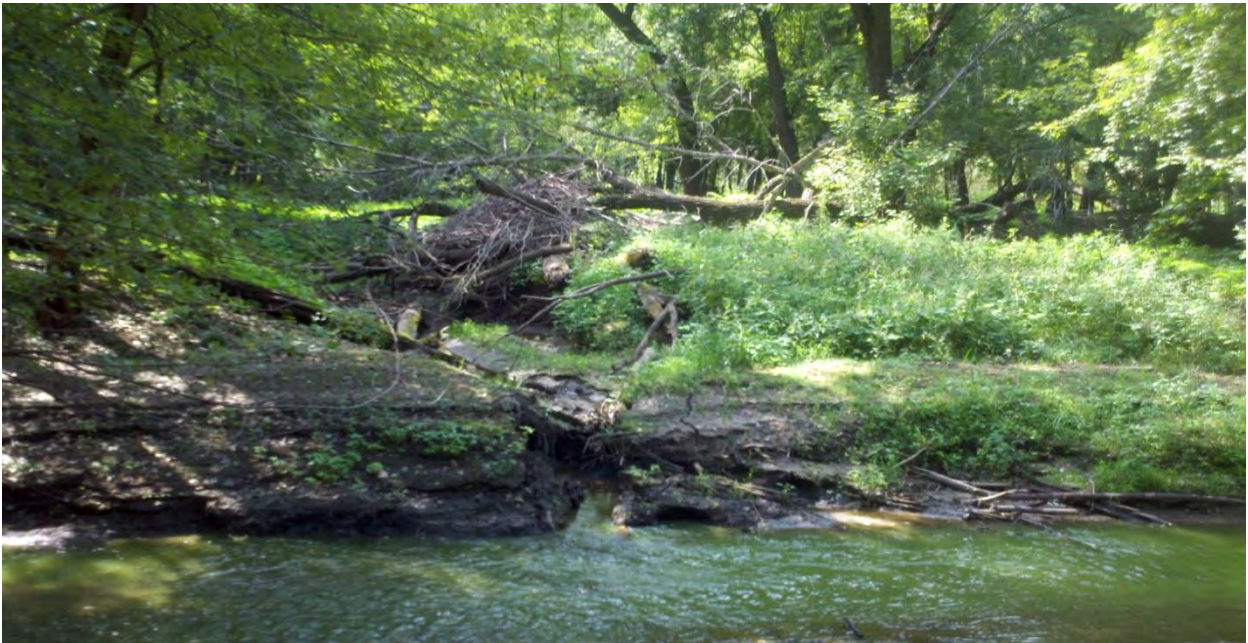
Photo 4. Carver Creek gully approximately 150 feet upstream of trail crossing
